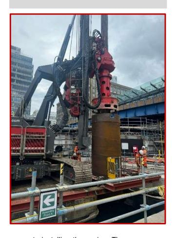
comes to installing the casing. The presence of the Lambeth granular formation and Thanet Sands has also meant that the piles were installed under polymer support fluid to maintain open shaft stability.
