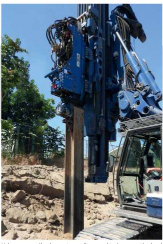
H-beam as a pile element are often used to improve the load bearing capacity of the ground.
