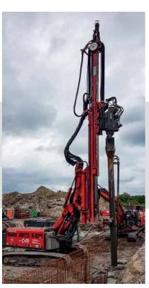
Displaceable soils are suitable for the installation of cast-in-situ full displacement piles.
