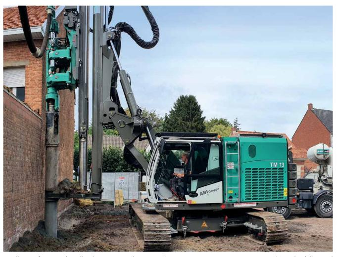
Installation of secant pile wall with a minimum distance to the existing structure using a VDW auger drive. The drilling and concreting is carried out in one continuous step, after drilling down concrete is pumped during withdrawal.
