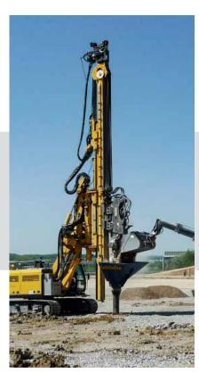
Increasing the load bearing capacity of the ground installing gravel piles.
