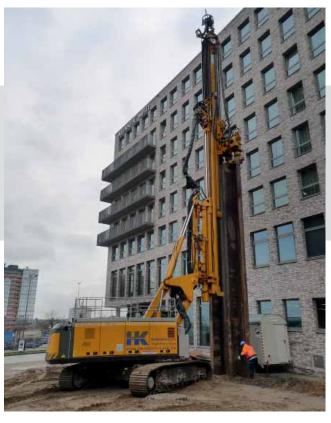
Static pressing directly in front of existing buildings. In some cases the soil must be loosened by pre-drilling before pressing.
