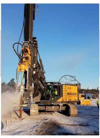
In hard, rocky soils down-the-hole hammers (DTH) are used for drilling.
