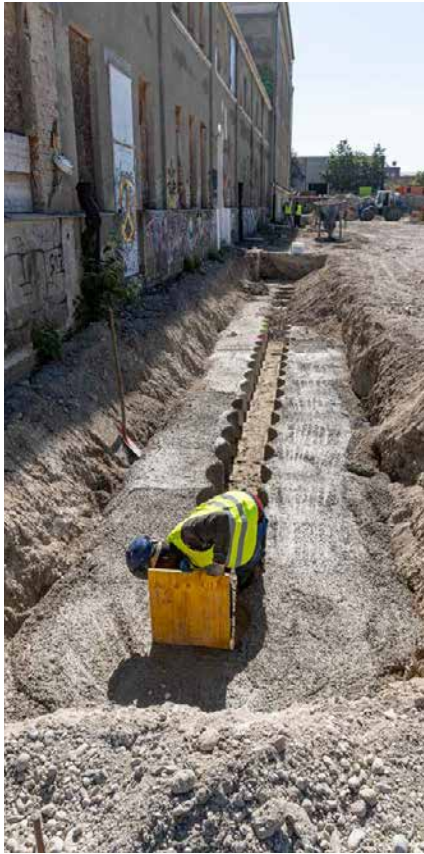
Photo: Template for a secant pile wall
