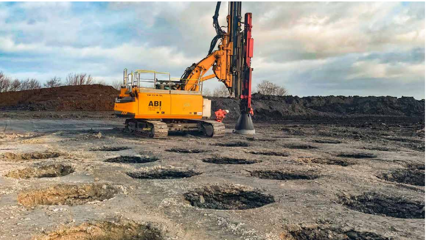
Photo: ABI MOBILRAM TM 13/16 SL with DELMAG diesel pile hammer D19-52 and compaction foot
