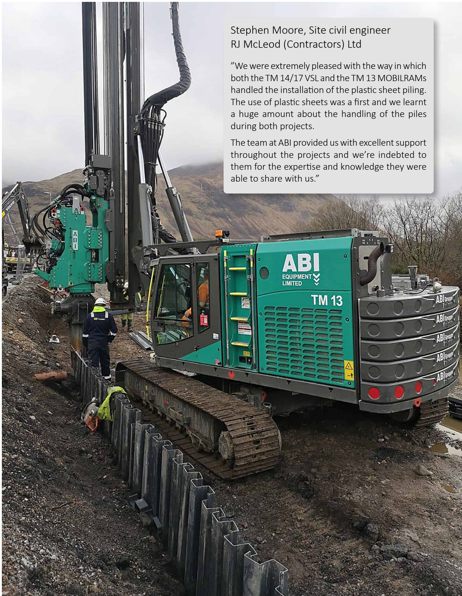
Photo: ABI MOBILRAM TM 13 while pile driving plastic sheet piles on the flood protection project at Caol and Lochside
