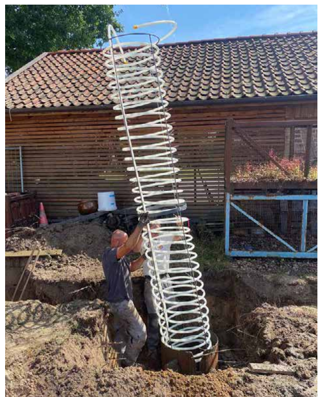
Photo: installation of geothermal probe in the cased bore hole
