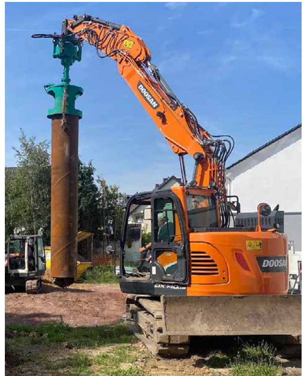
Photo: cased drilling with ABI excavator mounted auger drive BA 2200 and casing twister
