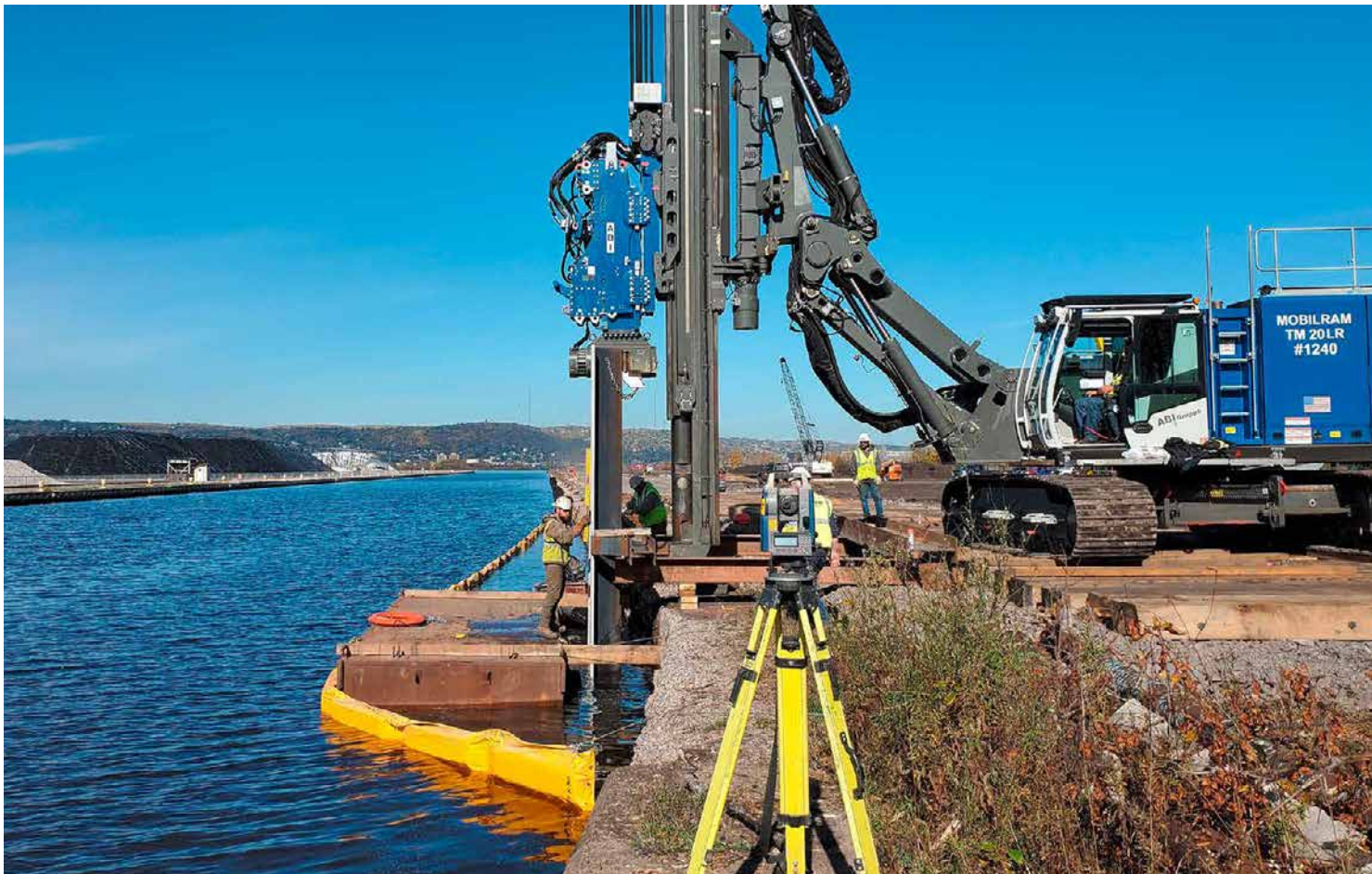
Photo: ABI MOBILRAM TM 20 LR with Vibrator MRZV 30VV on the St. Louis River, USA
