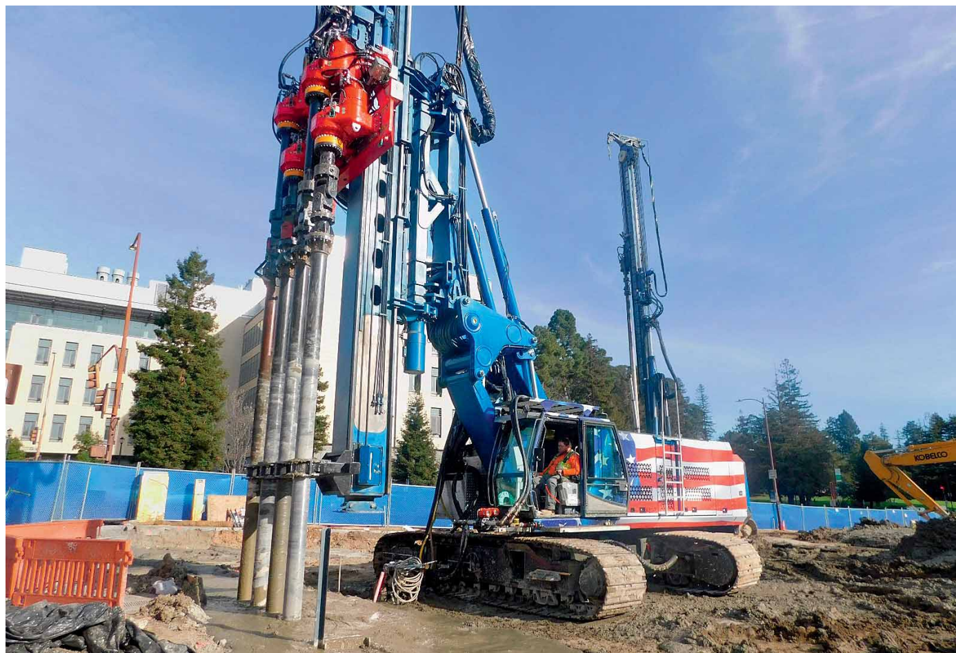
Photo: Quadmix TMBA 4-10000 with cardanic joints for easy assembly (above) Soil mixing works on a construction site in Berkeley, USA (below)
