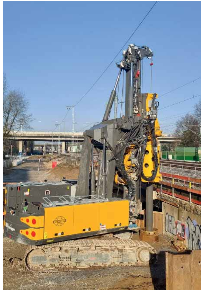
Photos: DELMAG drill rig RH 24/270 as short leader mast produced drilled piles in Kelly drilling process (above and below)
