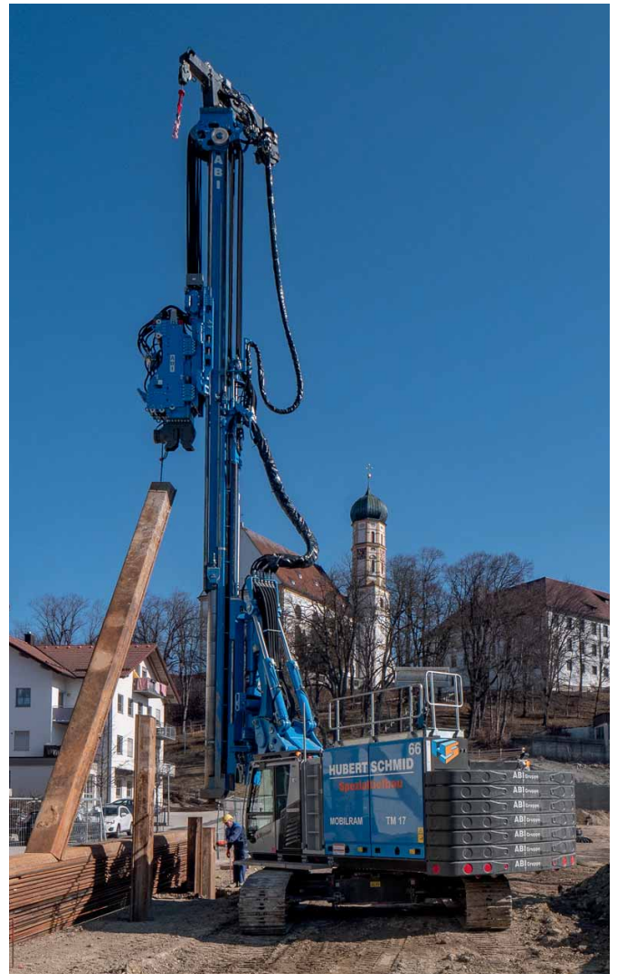
Photos: ABI MOBILRAM TM 17 with vibrator pile driving (right), Drill rig RH 12/140 birds eye view Kelly drilling (below) Source: Hubert Schmid GmbH
