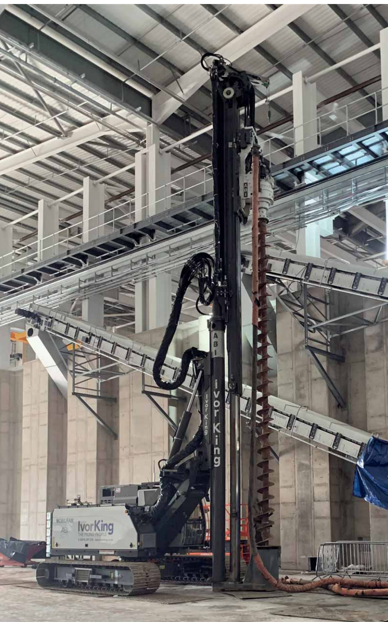
Photos: Job site of Ivor King Piling - TM 13 with auger drive MDBA (above) Finished king post wall inside the operational building (right)
