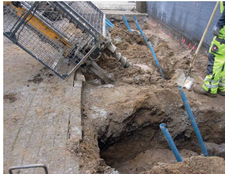
Photo: Inclination drilling with partial displacement auger for insertion of empty plastic tubes
