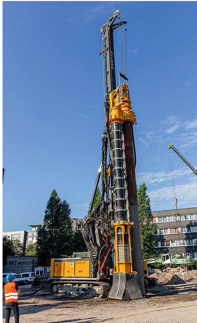
Photos: Pile production with VDW auger drive, the drill spoil is safely guided to the ground so that there is no danger to the construction site personnel
