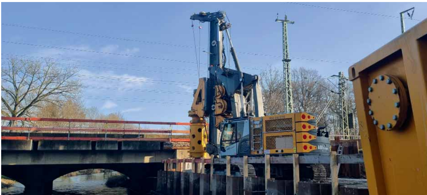
Photos: DELMAG drill rig RH 24/270 as short leader mast produced drilled piles in Kelly drilling process (above and below)
