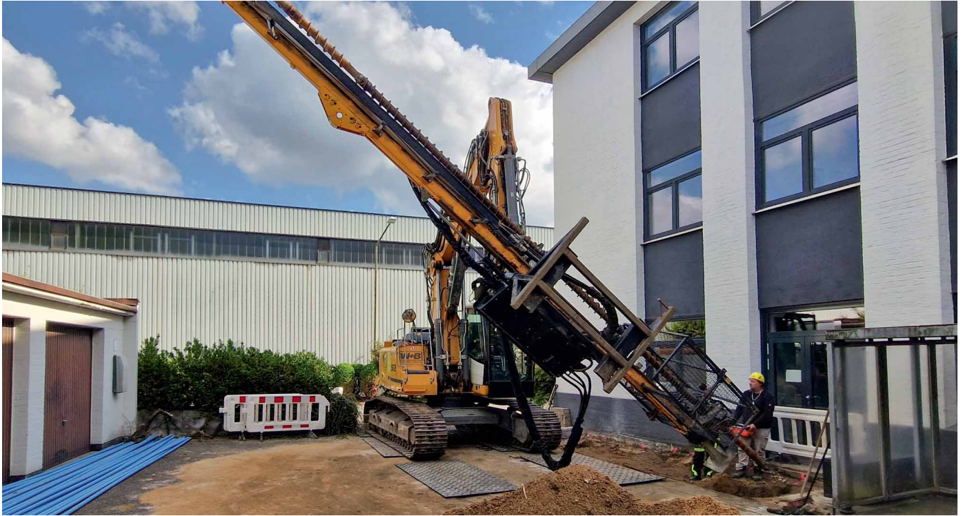
Photo: SPD excavator mounted drilling mast MD80
