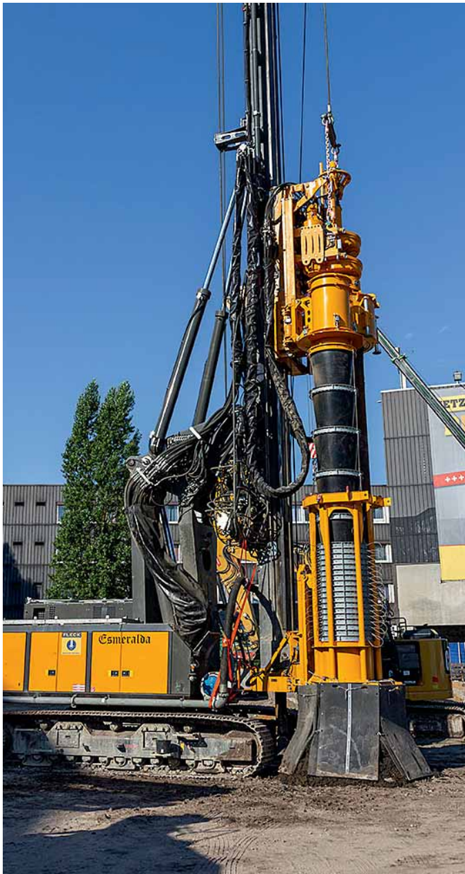
Photos: Pile production with VDW auger drive, the drill spoil is safely guided to the ground so that there is no danger to the construction site personnel
