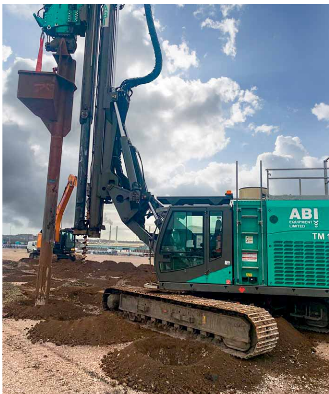
Photo: Job site of Trittech Ground Engineering Ltd - TM 13 with vibrator MRZV 12VV installing stone columns (above)
