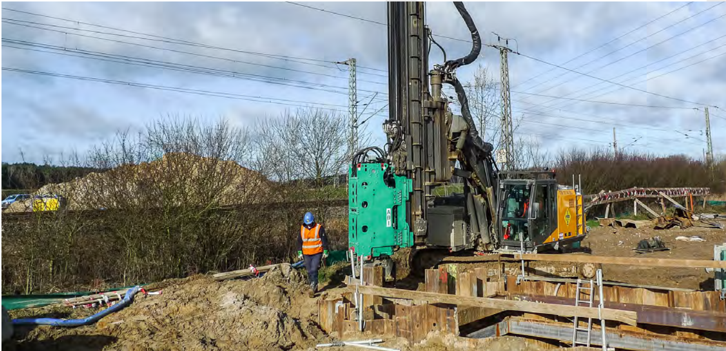
Photo (above and left): ABI MOBILRAM TM 11/14 SL with vibrator MRZV 16VV on a job site of the company Firma PRB near Anklam
