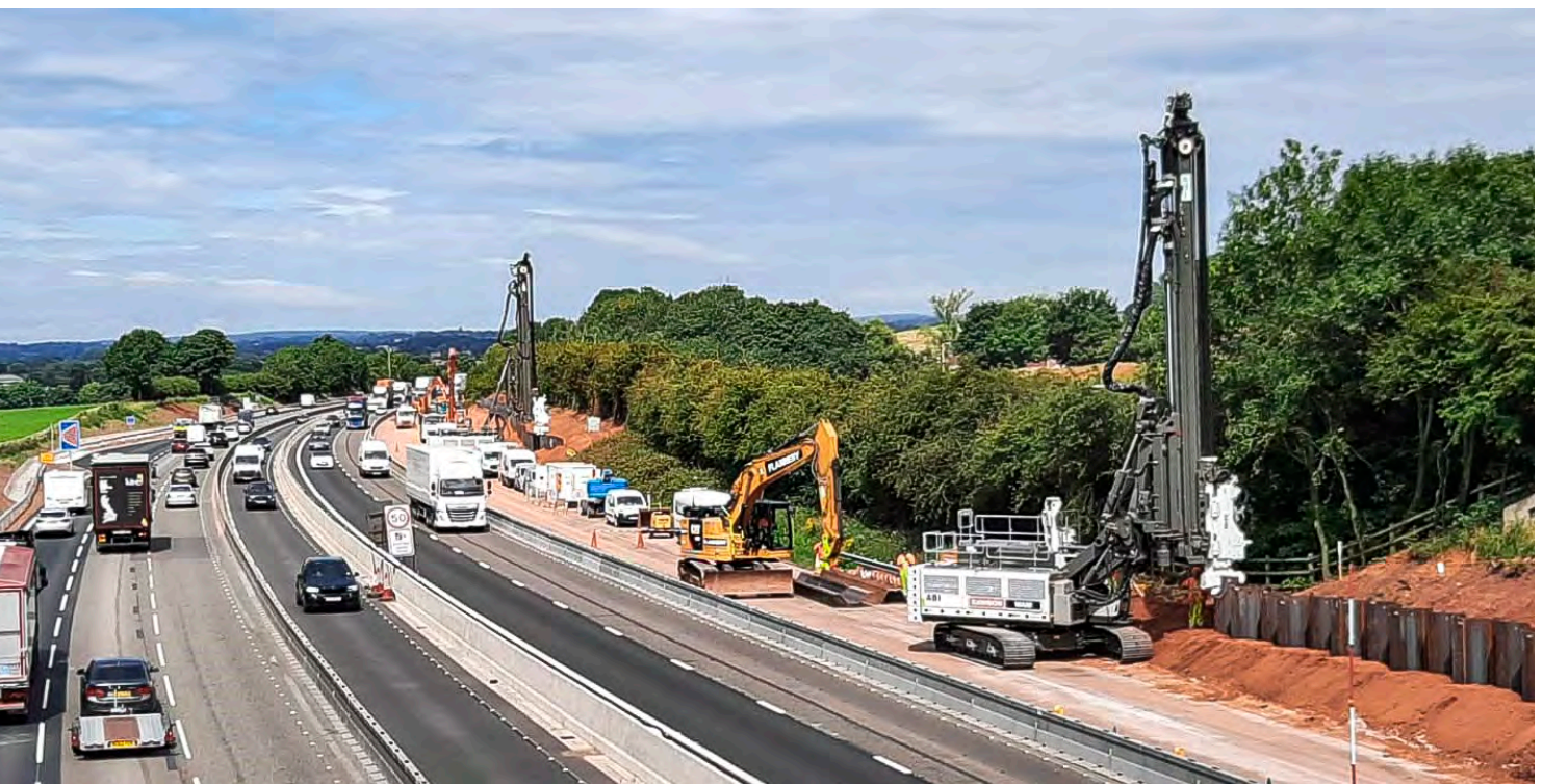
Photo: Two ABI MOBILRAM-Systems pile driving on the M6 motorway (TM 22 and TM 20)
