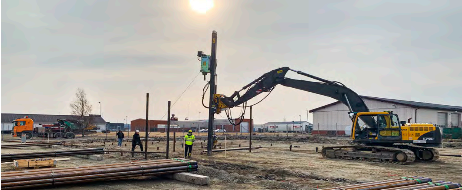
Photo: The Company's own personnel and machinery, in this case a PM85-EC290 piling rig, were used for the foundation works in Sala, Sweden
