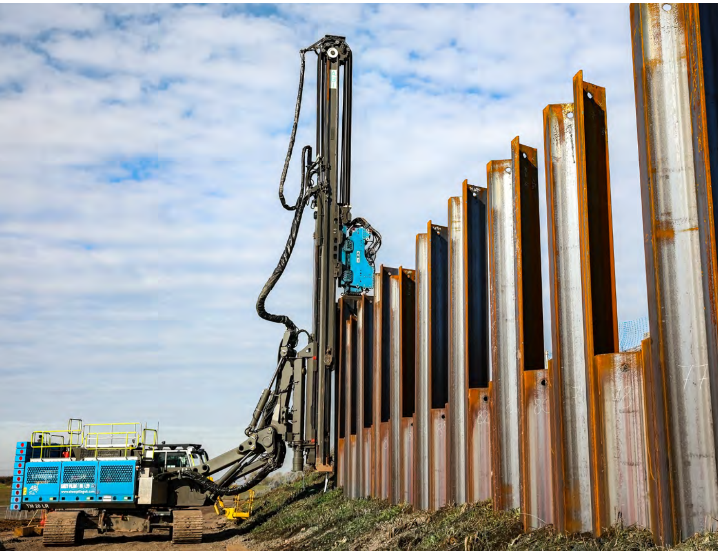
Photo: Credit: Sheet Piling (UK) Ltd - www.sheetpilinguk.com , Pile driving with ABI MOBILRAM TM 20 LR with extended reach
