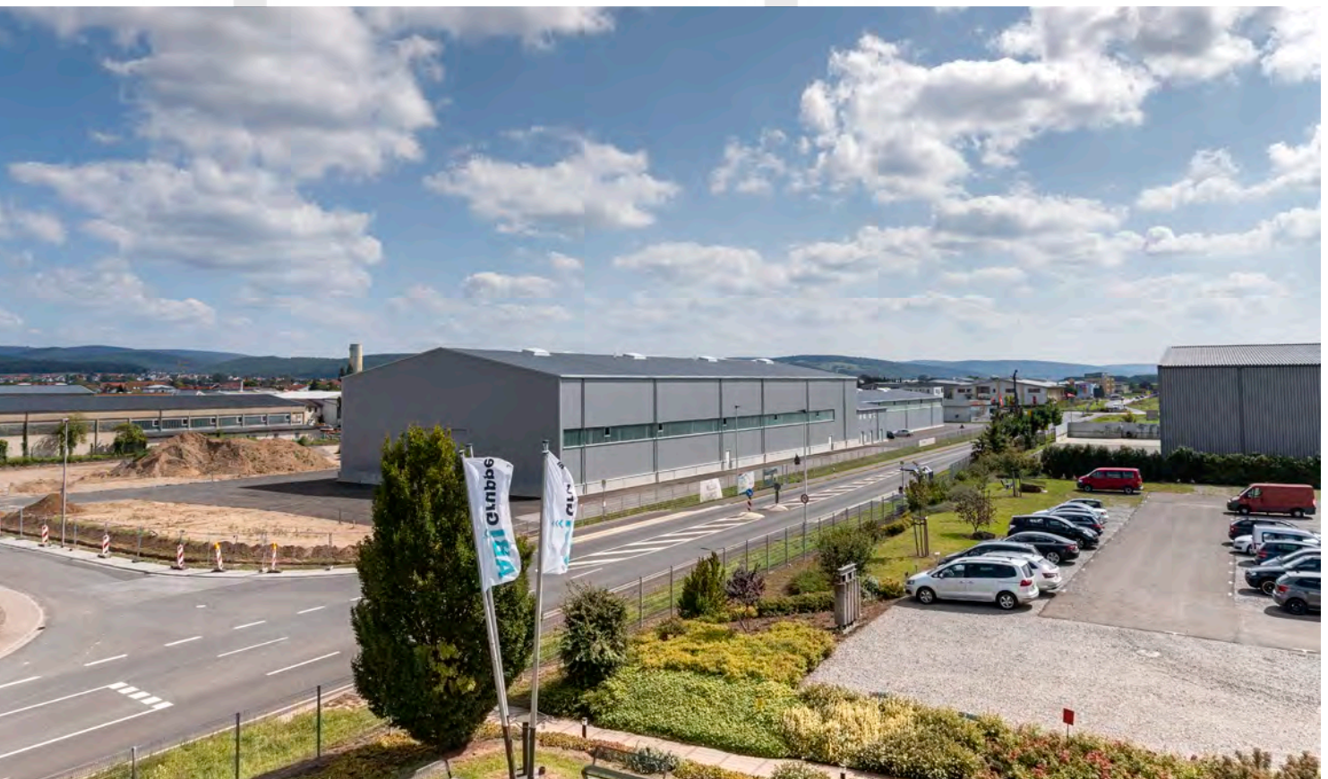
Photo: ABI premises at the Boschstraße 2 in Niedernberg, Germany with new halls mechanical production and welding shop
