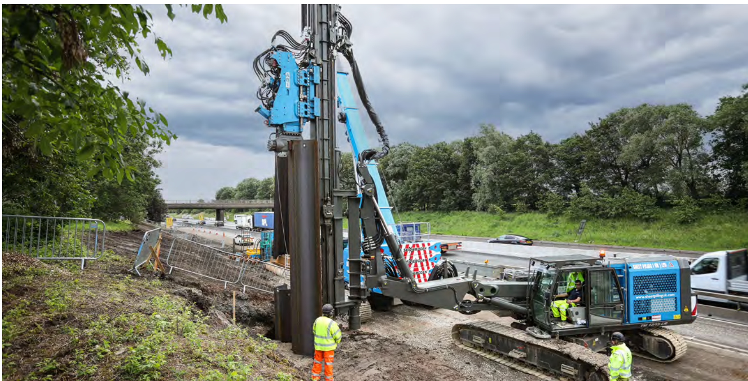
Photo: Credit - Sheet Piling (UK) Ltd - www.sheetpilinguk.com TM 12/15 H-LR with extended reach while pile driving with vibrator MRZV 20VV
