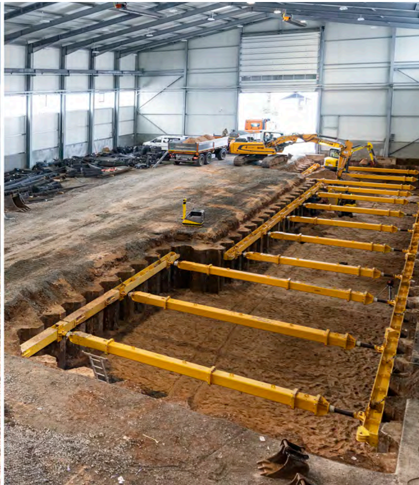
Photo: Driving steel sheet piles for the foundation of the future location of the CNC machine with an ABI MOBILRAM-System (left), excavation of the foundation in the almost finished hall (right)
