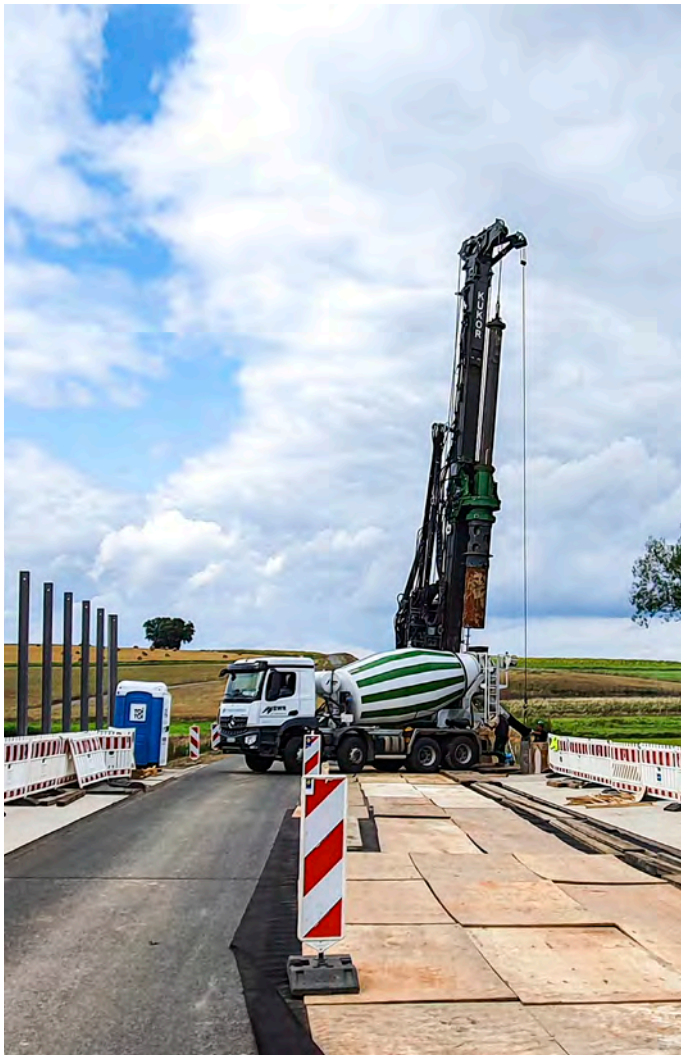
Photo: DELMAG drill rig RH 24/270 during concreting, the contractor pipe was lowered into the borehole with the auxiliary winch
