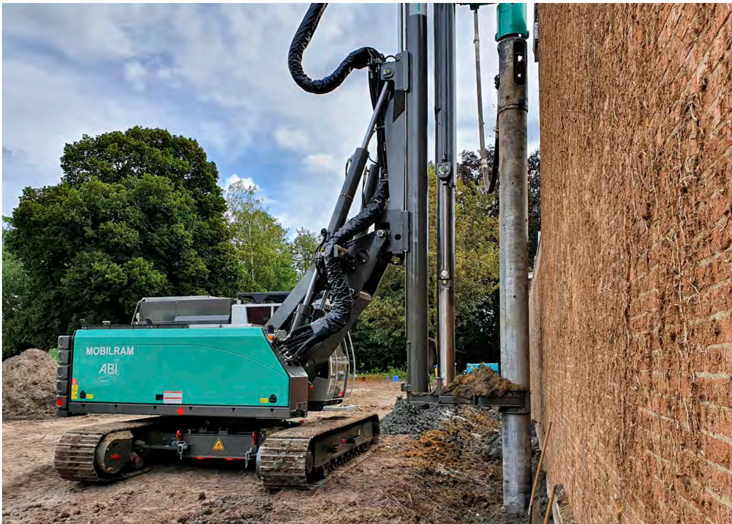
Photo: Maximum use of space, construction of a secant pile wall directly in front of an existing wall using the VDW method.
