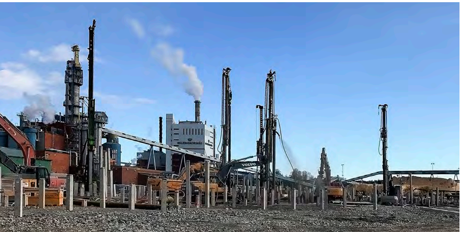
Photo: Foundation works in Grums (Sweden) for an extension of a paper mill with numerous SPD machines
