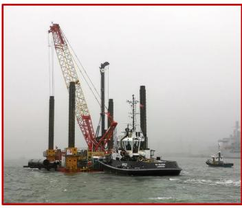
Two piles were required to be sunk, between which a 40m linkspan will land onto the new proposed pontoon structure. The pontoons will be fastened to the new piles to hold them in position. All work was carried out from Red7Marine's 400t jack-up barge sited just offshore in the tidal estuary.
