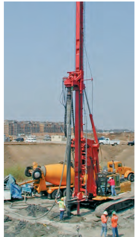
Full displacement drilling
