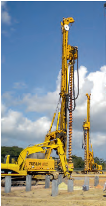
CFA drilling
