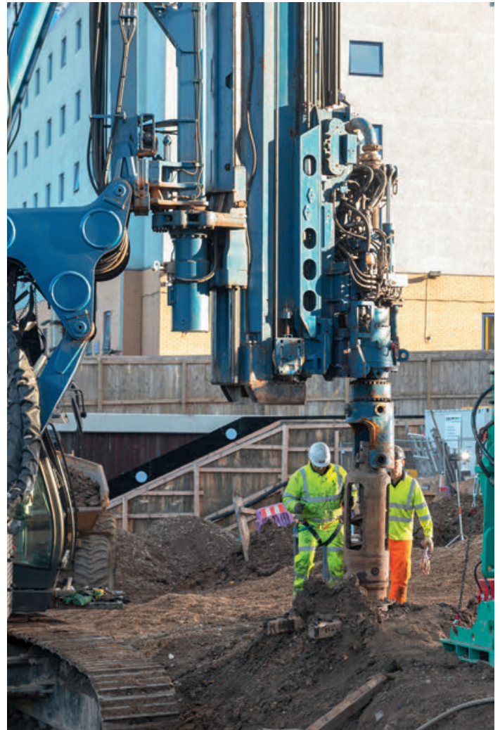
Photo: ABI MOBILRAM TM 22 with VDW equipment at the job site in North Acton
