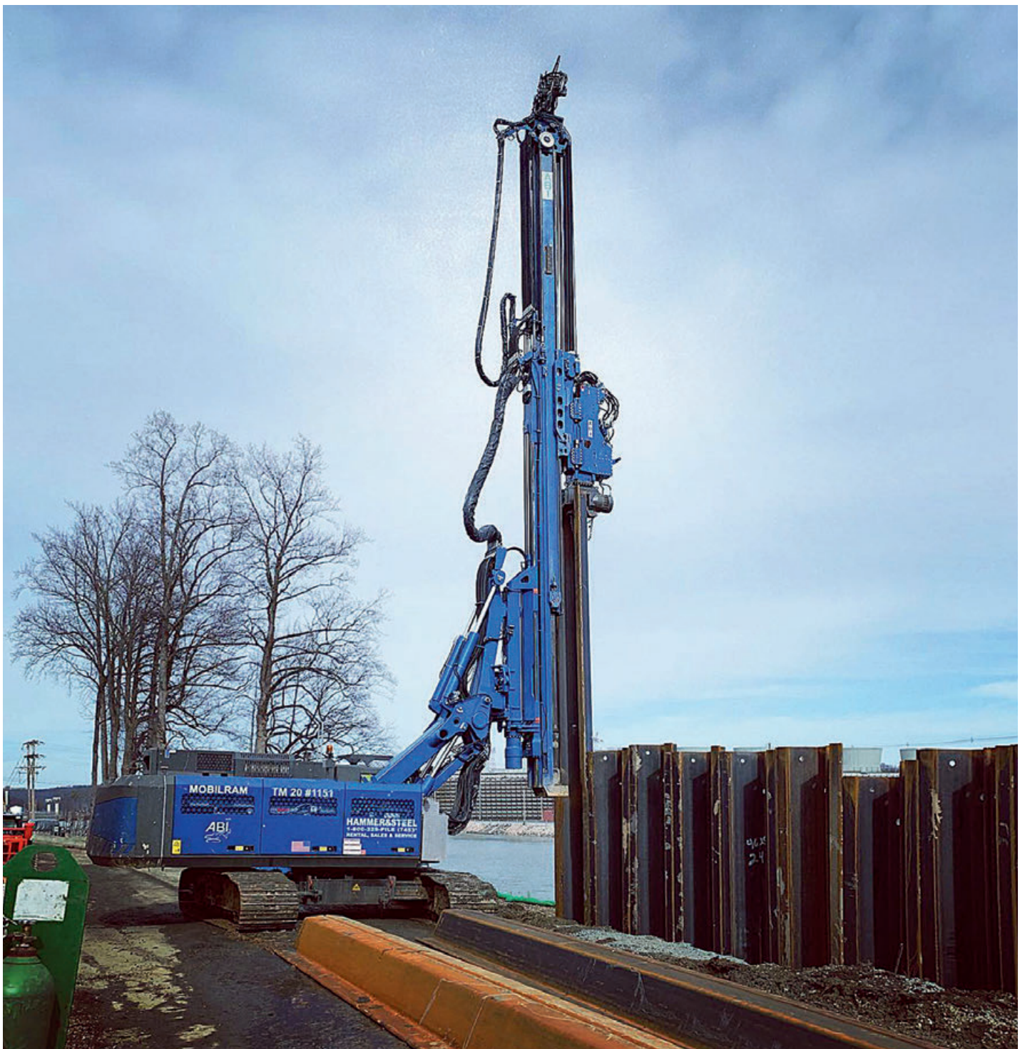
Photo: ABI MOBILRAM TM 20 while pile driving in Delta
