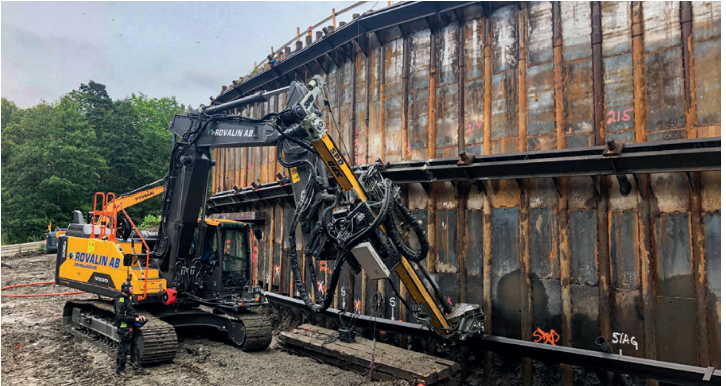
Photo: Drill mast DM55-EC250 of the company Rovalin while anchor drilling in Stockholm
