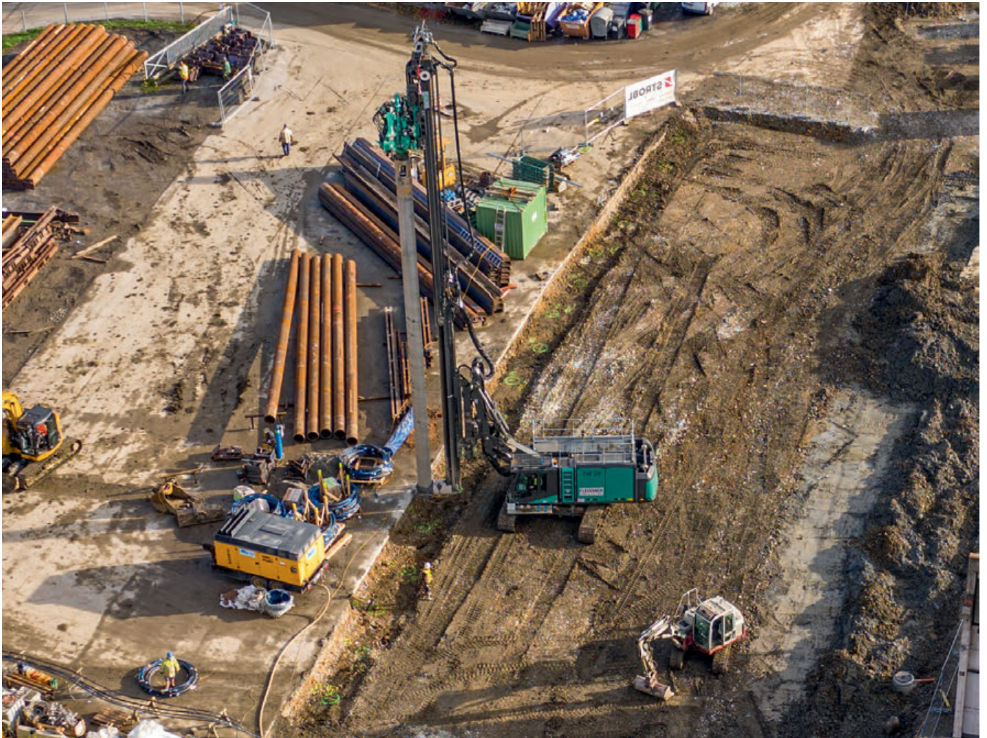
Photos: ABI MOBILRAM TM 20 with VDW equipment at the job site in Weiz (above), Finished shoring with sheet pile wall (below), TM 20 with double auger head system VDW 10050 and TM 14/17 SL with vibrator (left)
