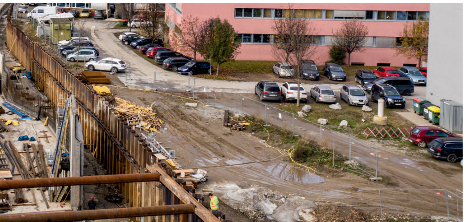
Photos: ABI MOBILRAM TM 20 with VDW equipment at the job site in Weiz (above), Finished shoring with sheet pile wall (below), TM 20 with double auger head system VDW 10050 and TM 14/17 SL with vibrator (left)
