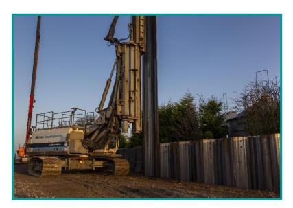
Using the MRZV 28VV and MRZV 17VV vibros, with their unique variable static moment / variable frequency capability, meant that it was possible to install the piles easily, efficiently and with least disturbance.
