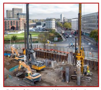
pile line of the correct width to suit the sheet pile sections. Accurate drilling position, and to some degree verticality, was greatly aided by the use of a purpose-built ground guide frame, designed by Dawson-WAM. Specially prepared 'cutting shoes' with a solid ring of carbide wear blocks ensured optimum coring efficiency was achieved whilst minimising tool wear and vibration.
