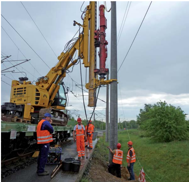
Picture: DELMAG G42 pipe clamp for holding pre-fabricated concrete masts
