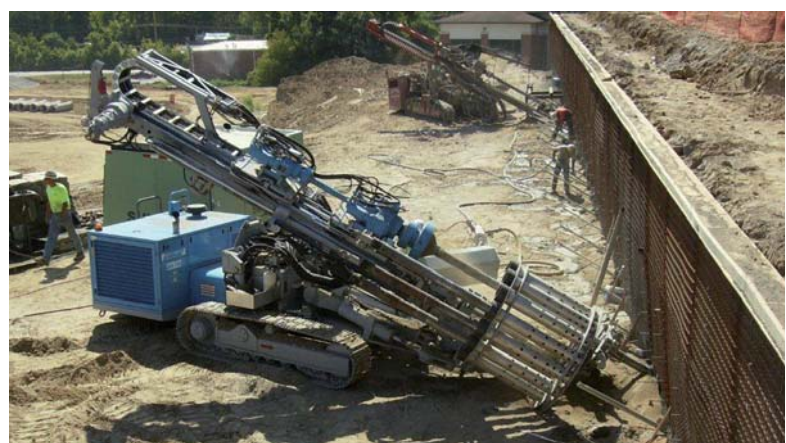
Picture: AN 150 with double head drilling unit DKB 2013 on the job site in St. Charles
