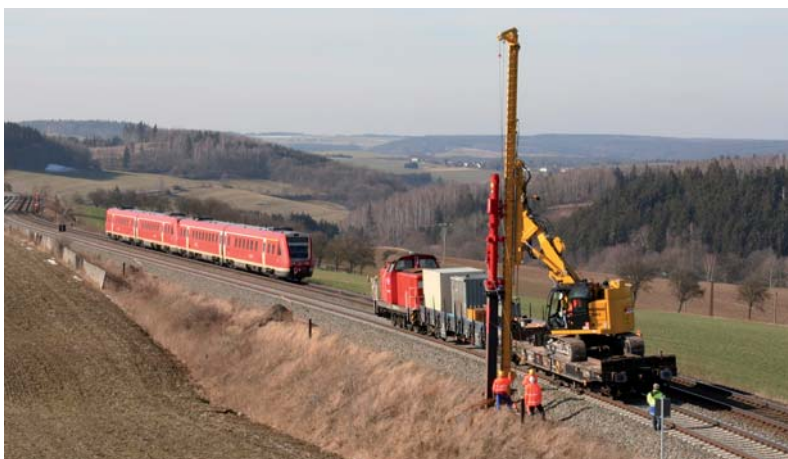
Picture: DELMAG G42 at the rail track between Plauen and Herlasgrün, the second track remained in service.
