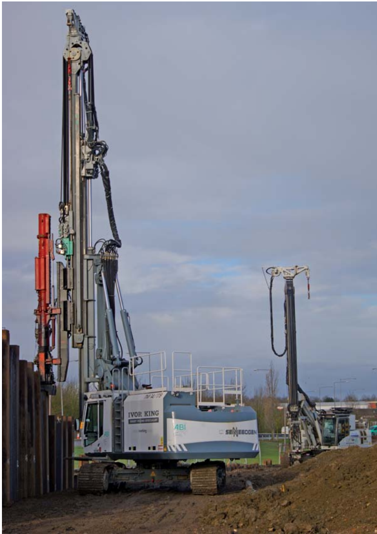
Picture: ABI MOBILRAM-System TM 14/17 B with DELMAG diesel pile hammer back-driving of steel sheet piles in Milton Keynes, England
