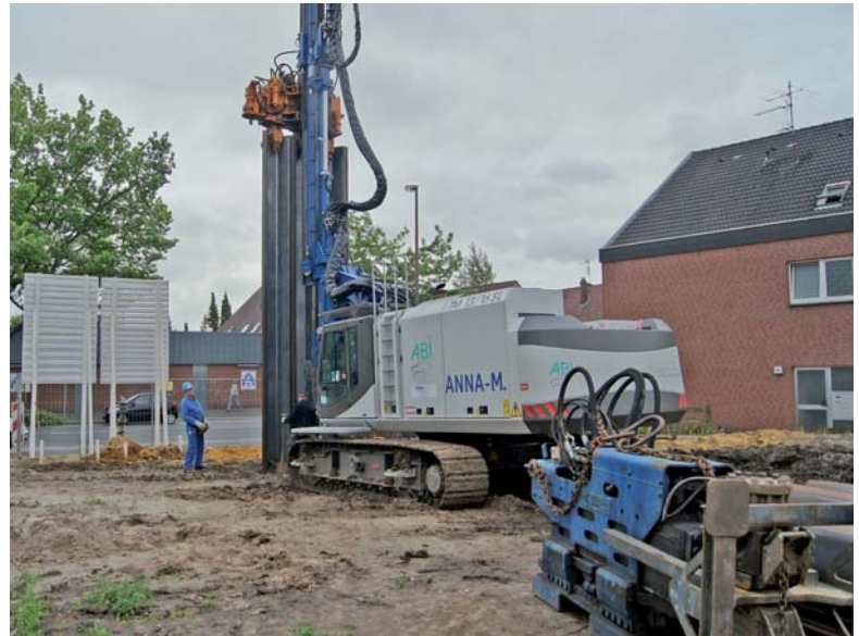
Picture: ABI MOBILRAM-System TM 13/16 SL with Hydro-Press-System in Oldenburg
