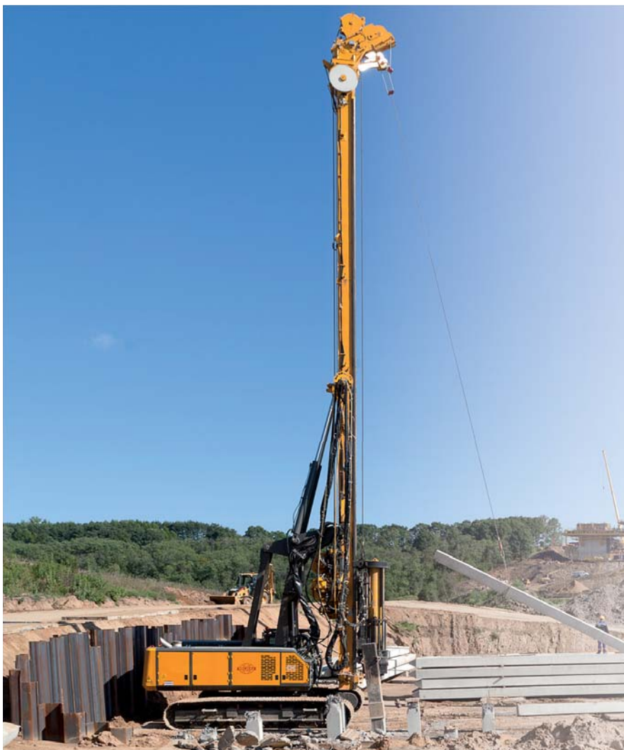
Picture: DELMAG drilling rig RH 34 SRH with SuperRAM 10000XL driving pre-fabricated concrete piles
