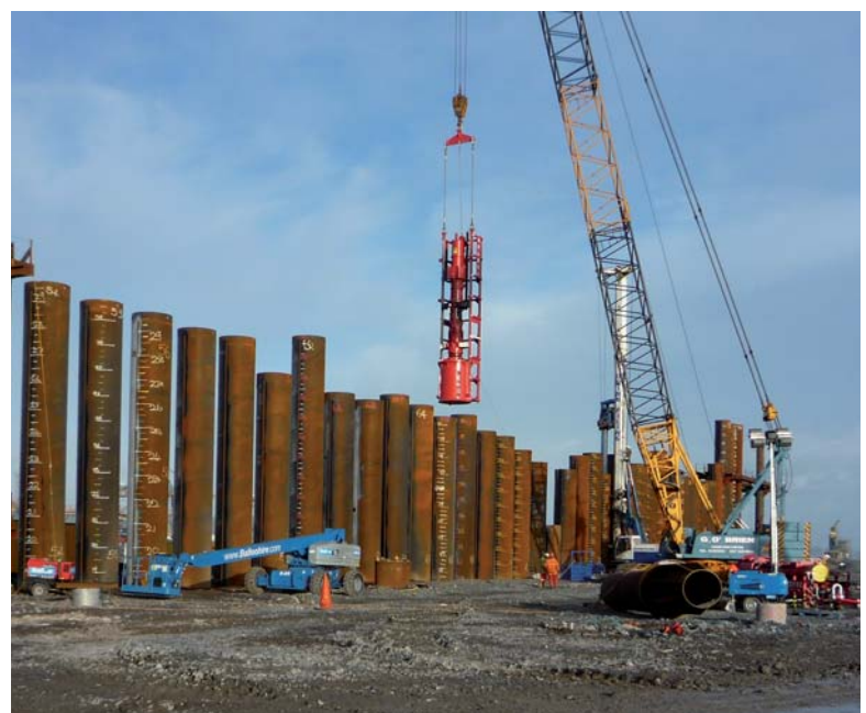
Picture: DELMAG diesel pile hammer D100 with rope suspended leader driving casings for the new quay in Belfast
