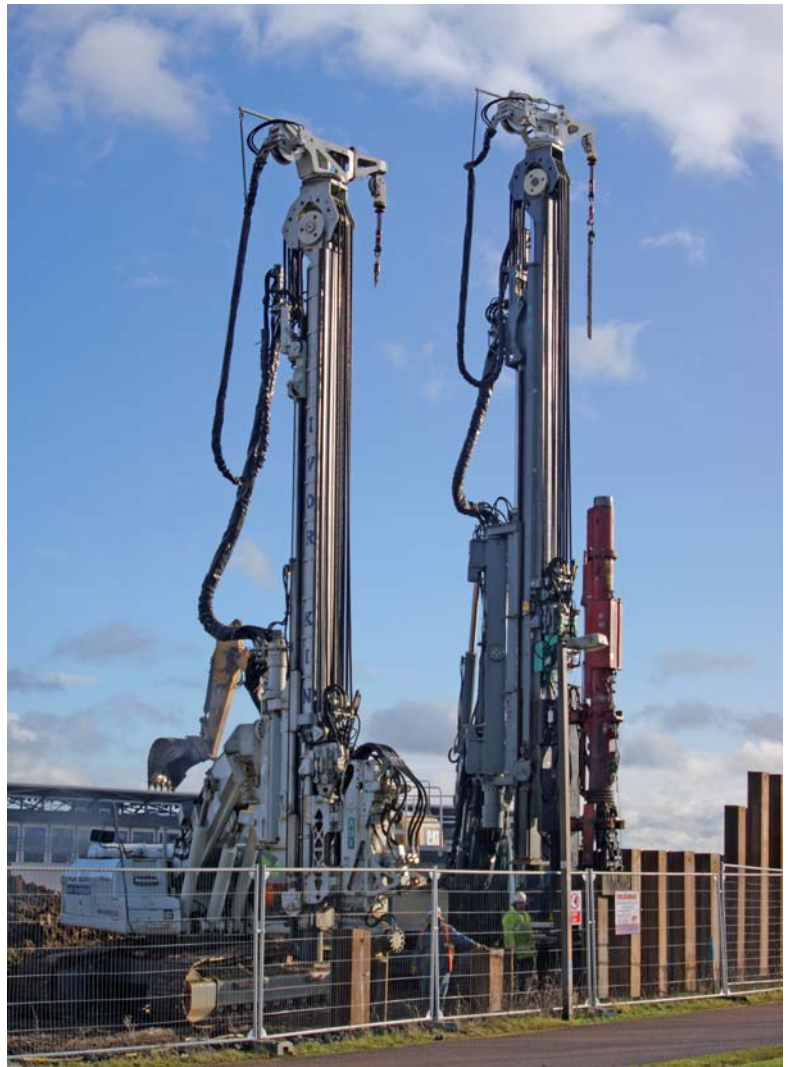
Picture: Working hand in hand Hand ABI MOBILRAM-System TM 14/17 B with DELMAG diesel pile hammer and TM 13/16 SL with vibrator MRZV 17VV
