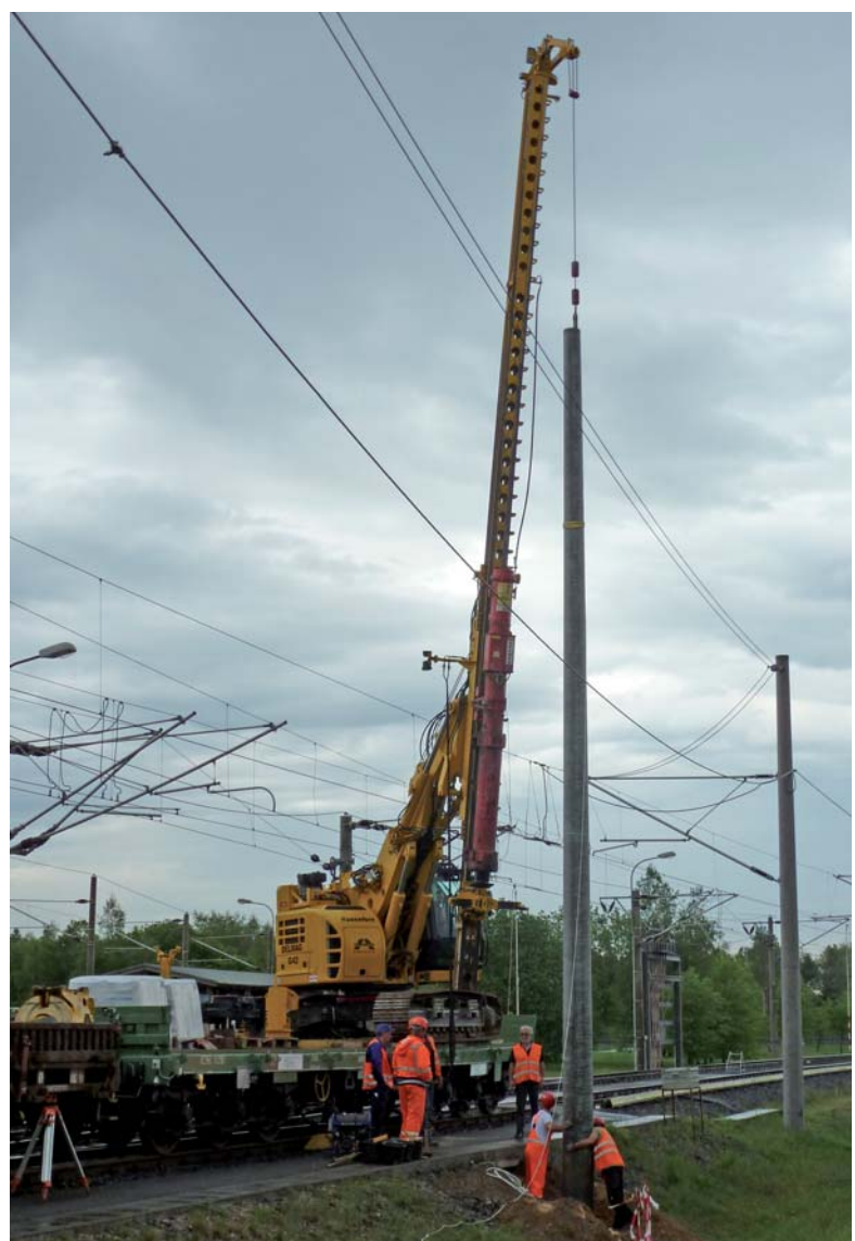
Picture: DELMAG G42, the pre-fabricated concrete masts are lifted and positioned with the auxiliary winch into the driven pipe
