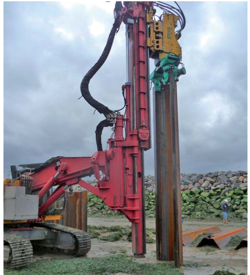
Picture: TM 11/14 equipped with vibrator and double clamp assembly for better guiding of the double sheet piles
