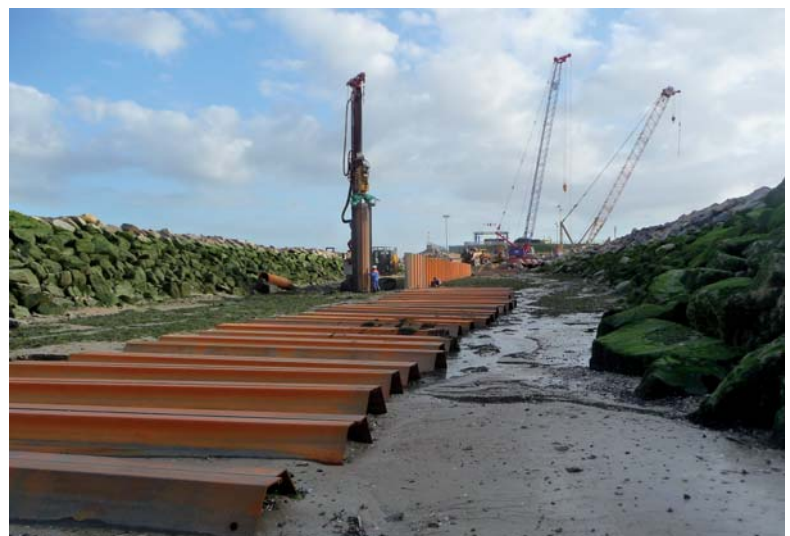
Picture: ABI MOBILRAM-System TM 11/14 at work in Ouistreham, the working times were determined by tides
