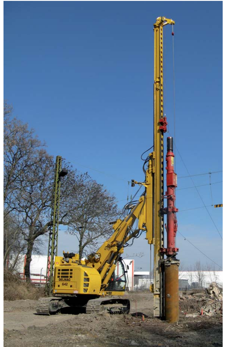
Picture: DELMAG G42 with diesel pile hammer D12-42
