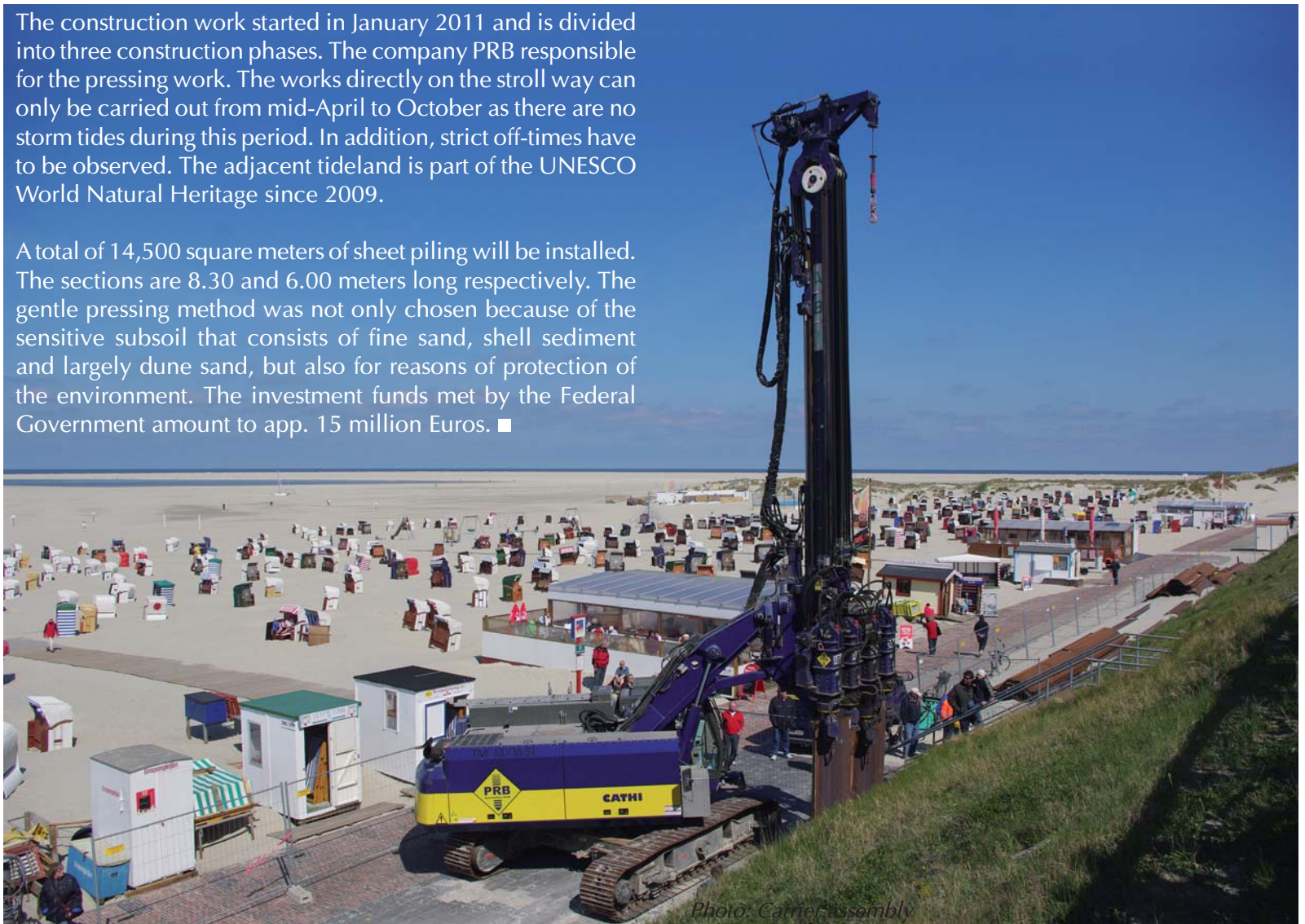
Photos: ABI MOBILRAM-System TM 13/16 with Hydro-Press-System HPZ on the jobsite at Isle Borkum
