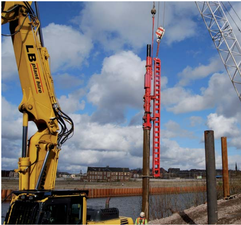
Photo: DELMAG diesel pile hammer D19 with swinging lead MS 1202 in Glasgow
