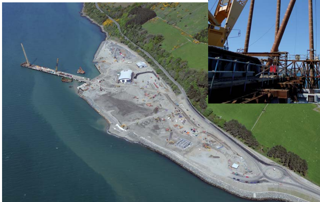
Photo: Aerial image of the job site at Loch Ryan, Detail: DELMAG diesel pile hammer D62 driving raked piles
