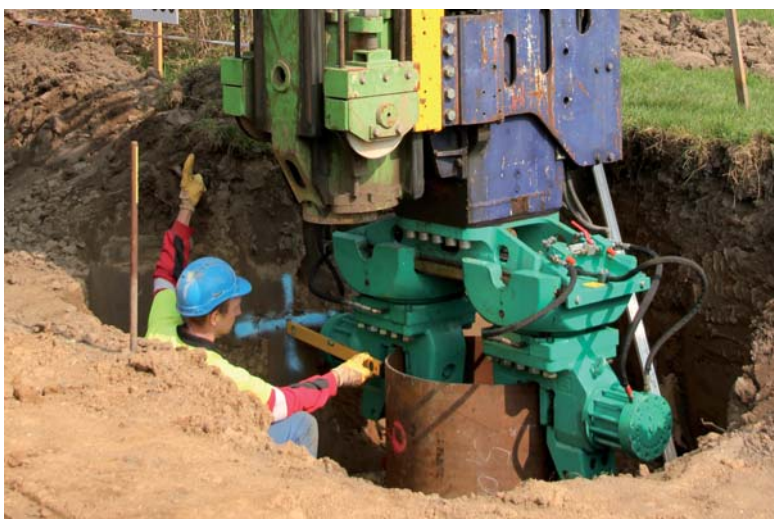
Photo (above): Combi clamp assebly MZK 800 Photo (right): ABI MOBILRAM-System TM 11/14 SL with Vibrator driving casings
