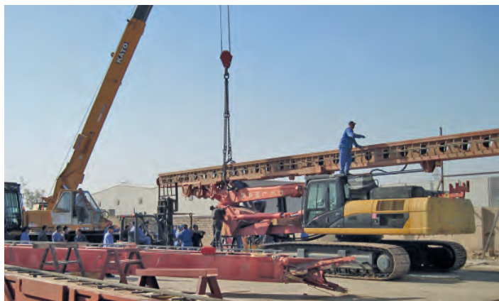
Photo: On site reassembly, leader mast and kinematics being connected with the new upper carriage
