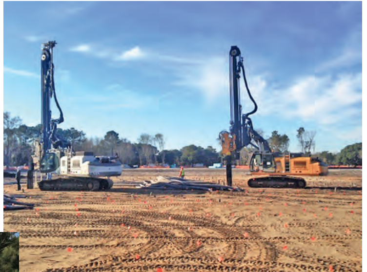
Photos: Two MOBILRAM-Systems TM 13/16 SL installing earthquake drains (above)
