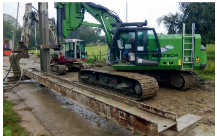
The telescopic leader mast with vibrator MRZV 17VV installing diaphragm wall (bottom and left)
