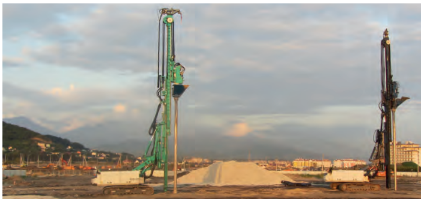
Photos: Large construction site in Sochi with two ABI machines installing stone columns
