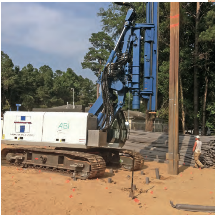
Photos: Two MOBILRAM-Systems TM 13/16 SL installing earthquake drains (above)
