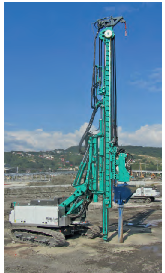
Photos: Large construction site in Sochi with two ABI machines installing stone columns
