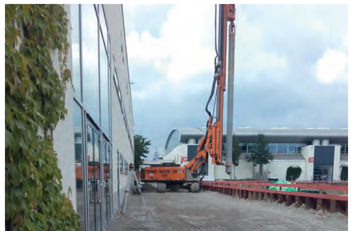
Photo: ABI MOBILRAM TM 17 was also used for the installation of concrete piles with VDW auger drive
