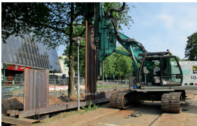
Photo: Steel sheet piles are driven into the ground using a guiding for exact positioning and accurate sheet pile wall alignment
