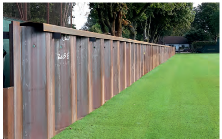
Photo: Finished sheet pile wall with top profile
