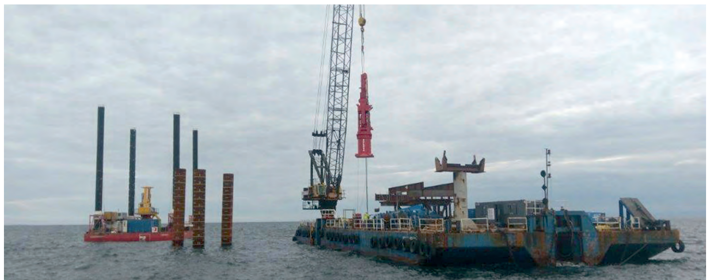
Photos: DELMAG diesel pile hammer D100-13 with rope suspended lead while driving (above). The diesel pile hammer is positioned with a crane on the ponton. (below)
