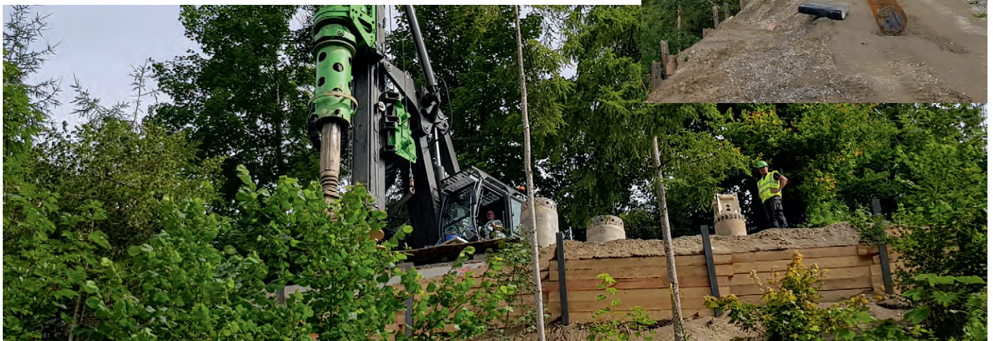
Photos: DELMAG drill rig RH 18/200 of the company D&K Spezialtiefbau at the job site in the municipality of Wolfegg (above), Photo: D&K Spezialtiefbau
