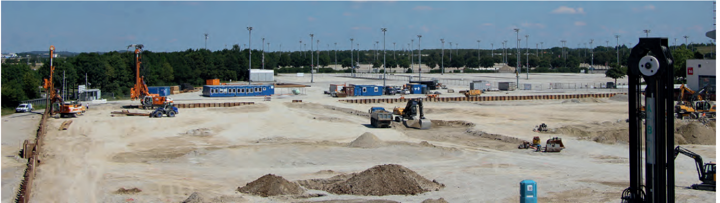
Photo: Exhibition grounds in Munich Riem at the beginning of the construction works
