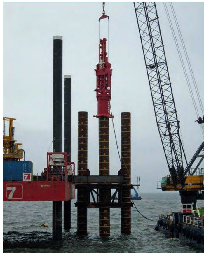
Photos: DELMAG diesel pile hammer D100-13 with rope suspended lead while driving (above). The diesel pile hammer is positioned with a crane on the ponton. (below)
