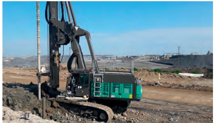
Photo: RH 30 at the job site on the link road to Istanbul's new airport installing mixed piles
