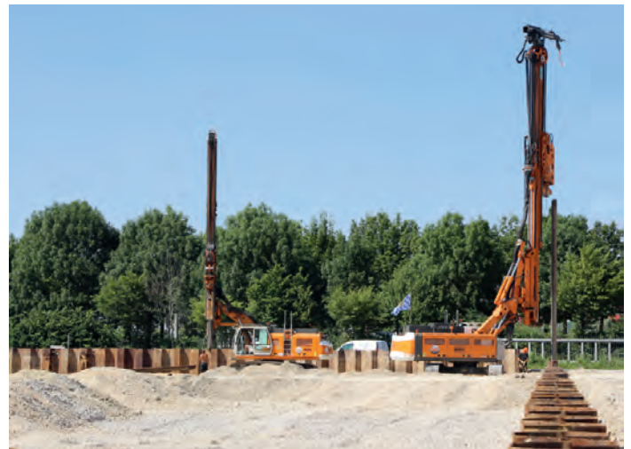
Photo: ABI MOBILRAM TM 17 and TM 14/17 SL while driving sheet piles for excavation support
