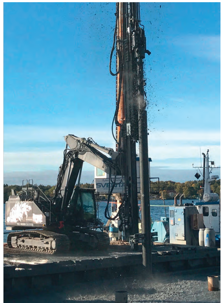
Photo: Telescopic drilling mast DT 145-EC300 with DTH hammer while drilling on the island of Lidingö, Sweden, Photo: SPD AB
