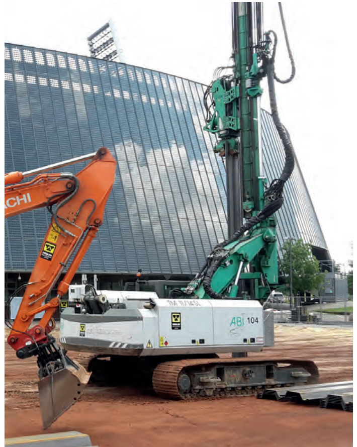
Photo: ABI MOBILRAM TM 11/14 SL with adjustable vibrator MRZV 17VV at Weser-Stadion
