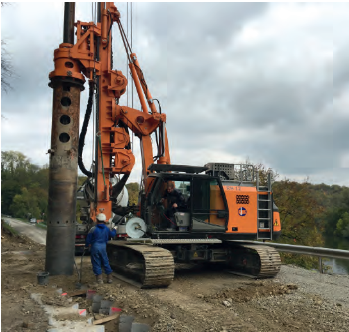
Photo: DELMAG drill rig RH 12 while Kelly drilling at the Neckar (Photo: GBS)
