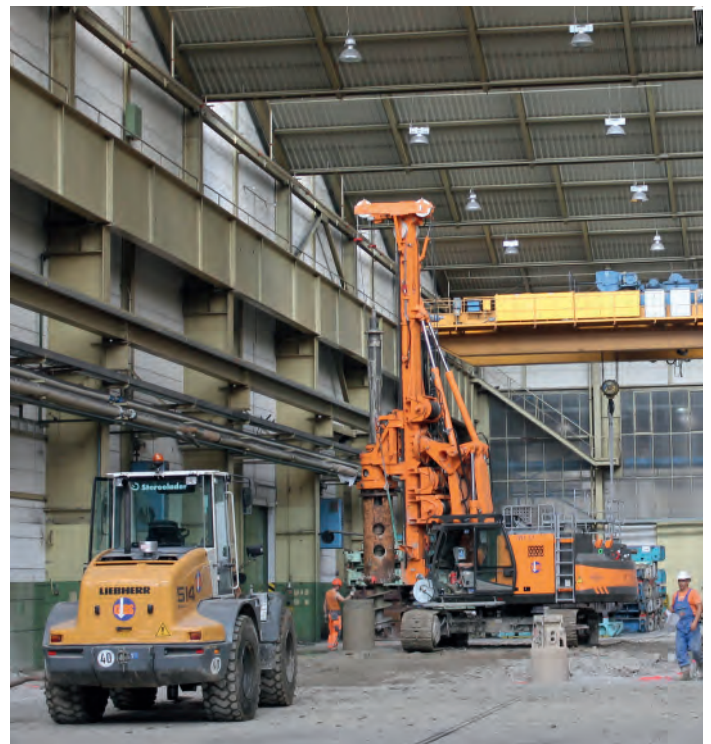
Photo: DELMAG drill rig RH 12 in a short leader mast version while Kelly drilling in a production hall (Photo: GBS)
