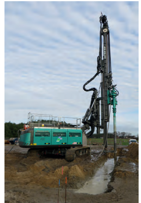
Photo: ABI MOBILRAM TM 14/17 V of the company M-TEC with Twinmix auger drive while soilmixing (above and below)
