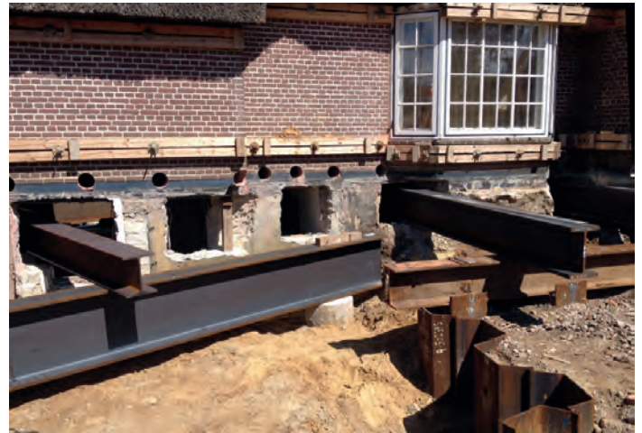
Photo: Holding structure made of steel beams, concrete piles and steel sheet piles
