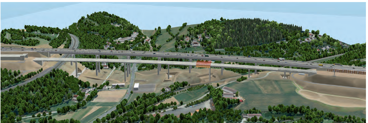
Graphics: A construction phase at the Heidingsfeld Viaduct © V-KON.media GmbH
