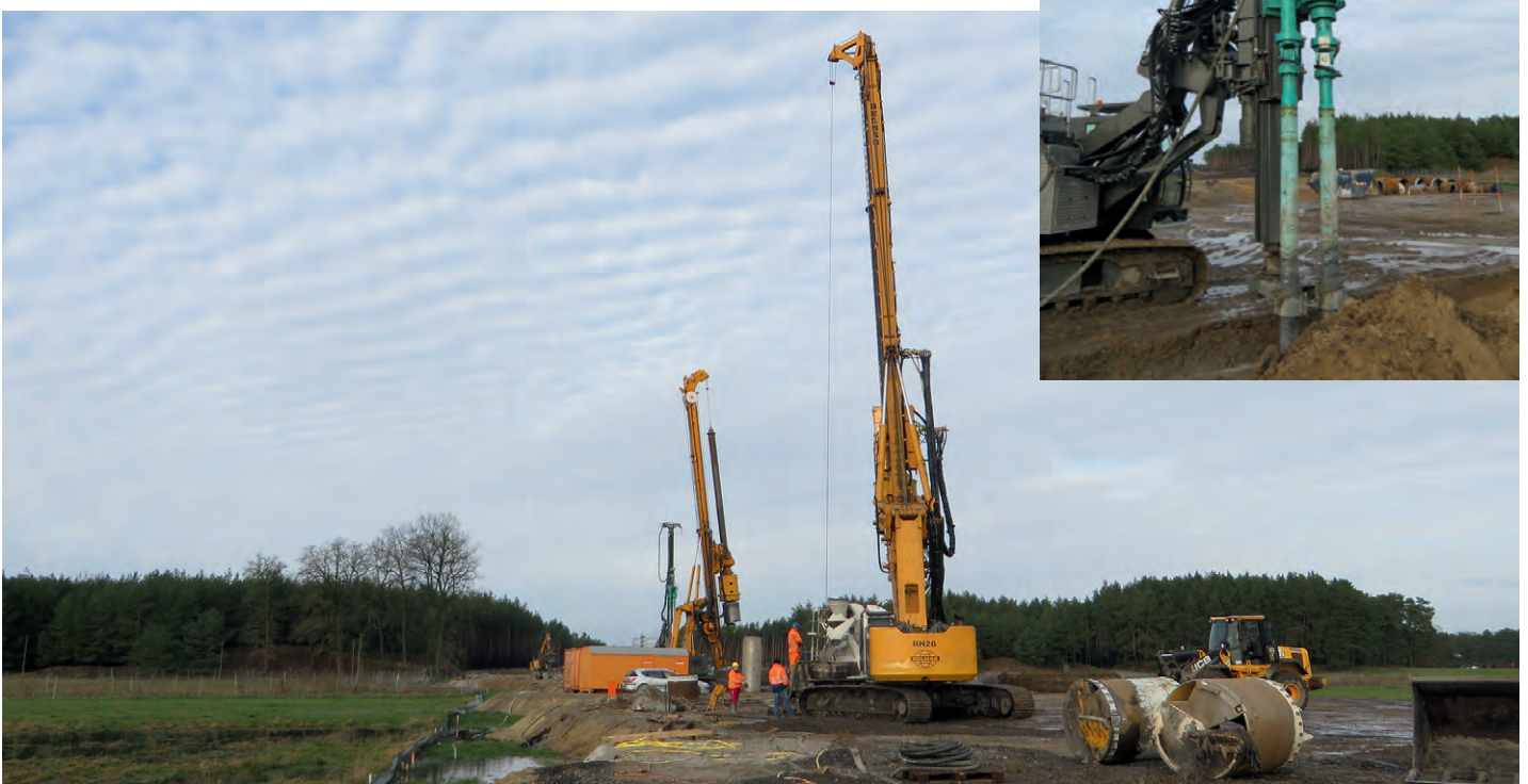
Photo: DELMAG drill rig RH 28 and RH 34 of the company Fleck while installing foundation piles
