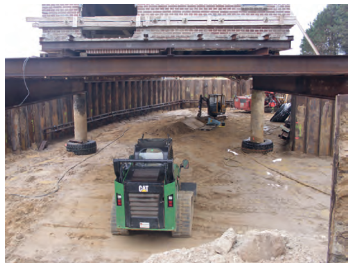
Photo: The basement is demolished, the building hovers
