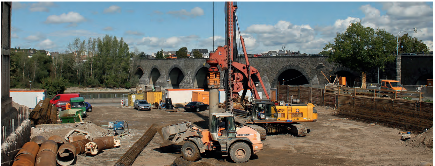
Photo: DELMAG drill rig RH 32 while installing foundation piles in Koblenz (Photo: GBS)
