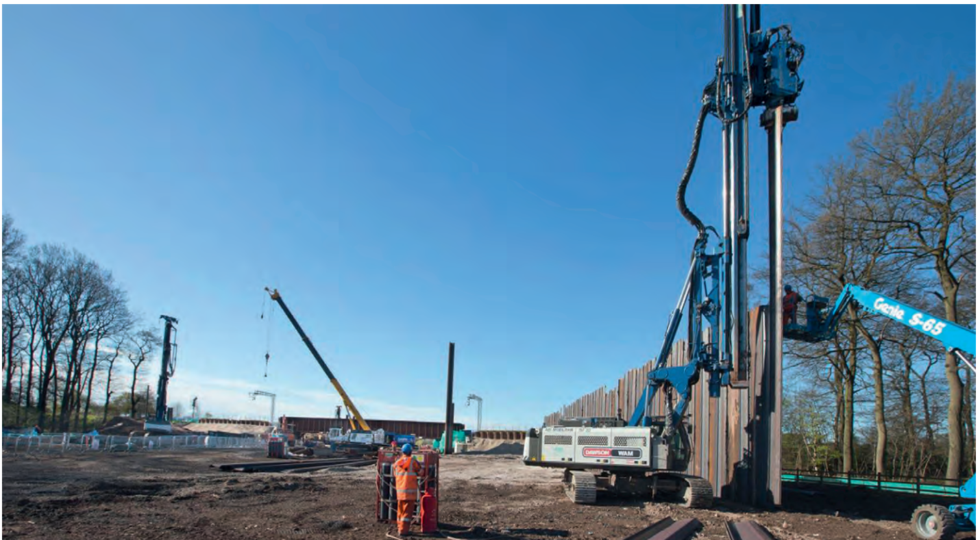
Photo: ABI MOBILRAM TM 22 installing jagged wall in Crewe
