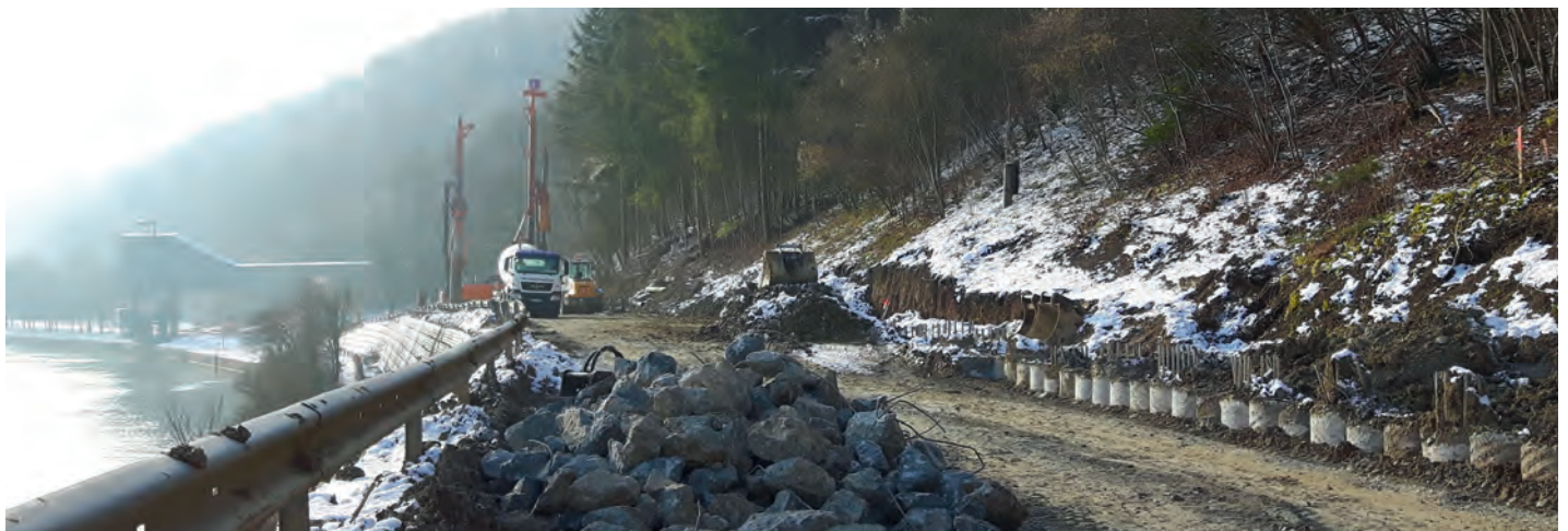
Photo: DELMAG drill rig RH 12 and RH 16 of the company GBS while Kelly drilling at the Neckar (Photo: GBS)
