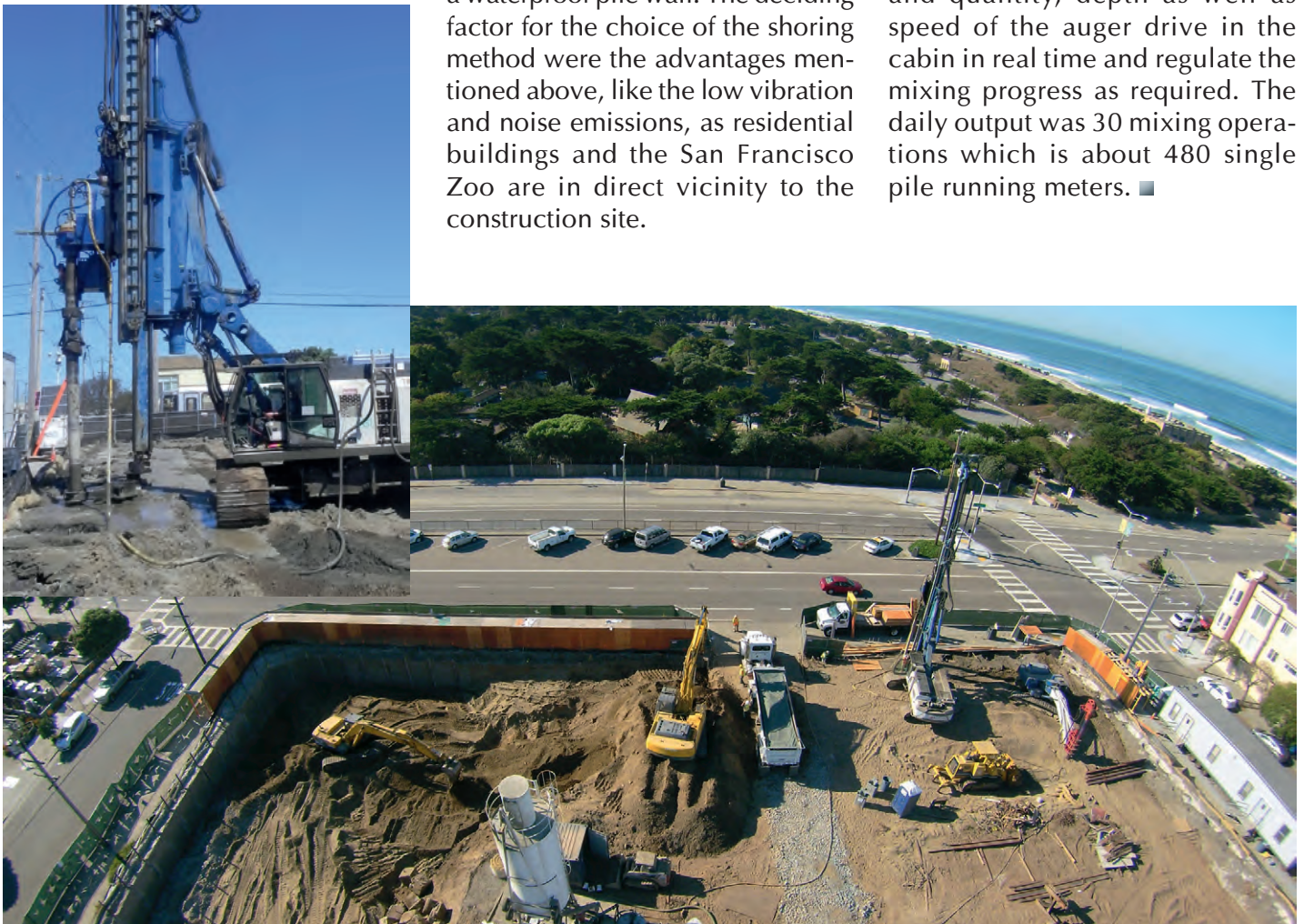
Photos: ABI MOBILRAM TM 18/22 B while installing the mixed piles
