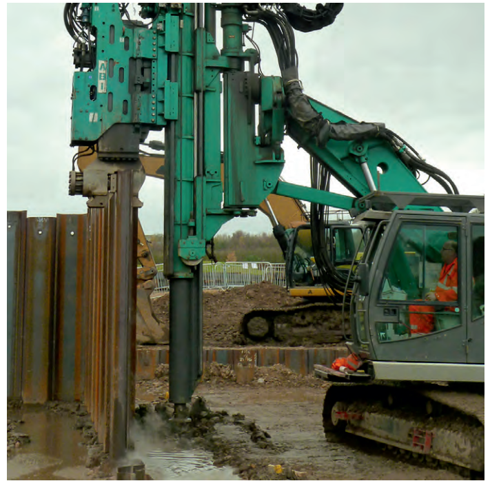
Photo: ABI MOBILRAM TM 13/16 while pile driving in Bishop Auckland
