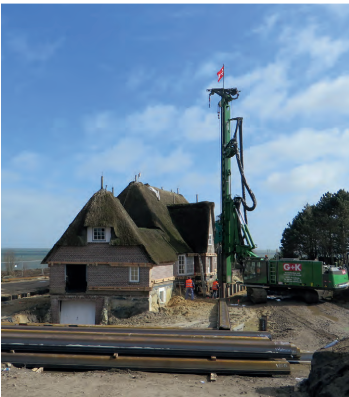
Photo: ABI MOBILRAM SM 12/16 with vibrator MRZV 20VV driving steel sheet piles
