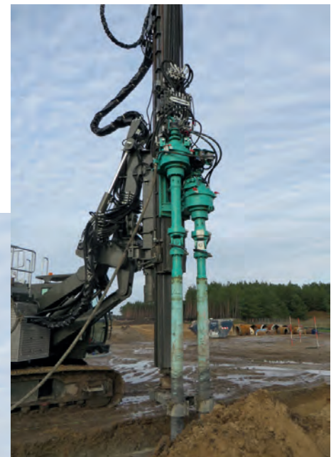
Photo: ABI MOBILRAM TM 14/17 V of the company M-TEC with Twinmix auger drive while soilmixing (above and below)
