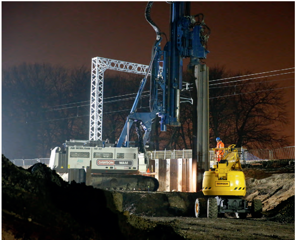
Photo: ABI MOBILRAM TM 22 with vibrator MRZV 30VV working during the night shift in Crewe
