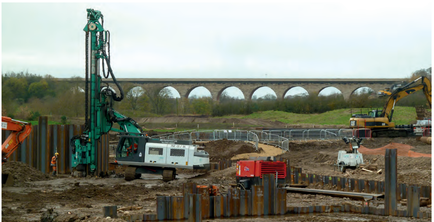
Photo: ABI MOBILRAM TM 13/16 while pile driving in Bishop Auckland
