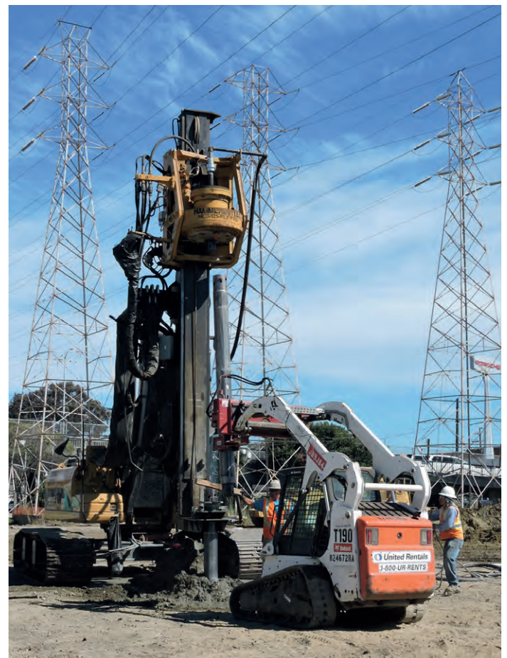
Photos: DELMAG drill rig RH 12 in short leader mast version while soil mixing
