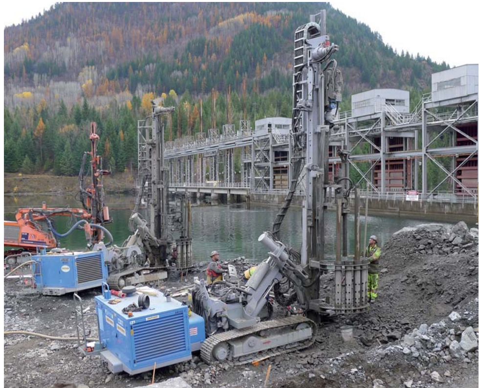
Photo: Drilling blast holes at the construction site of Waneta Dam in Canada
