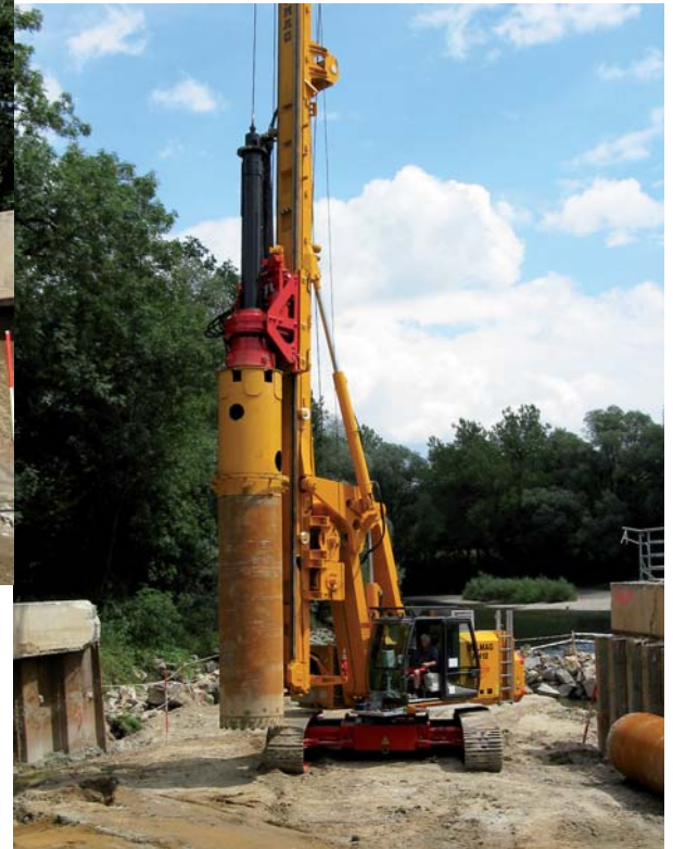
Photos: Replacing soils in Pillhofen at construction site of a new hydroelectric power plant
