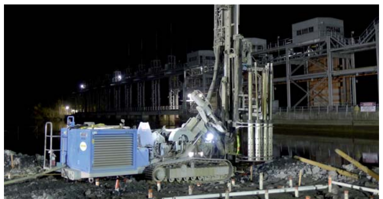
Photo: Working in spotlight, AN 150 while drilling at Waneta Dam during late shift
