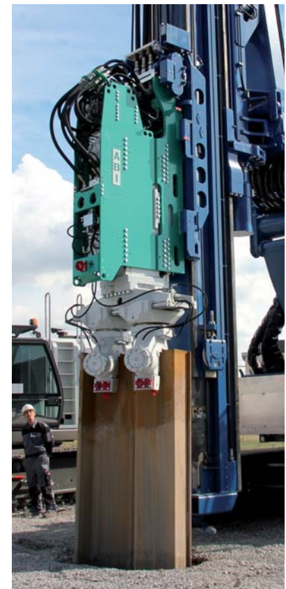
Photo: Vibrator MRZV 28VV with combi clamp assembly MZK 1250 at a double U sheet pile
