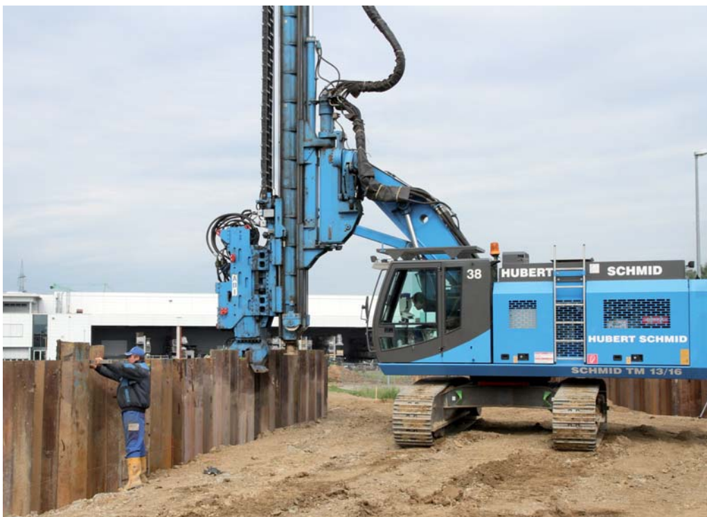
Photo: Telescopic leader mast TM 13/16 working on company site of Sennebogen in Straubing
