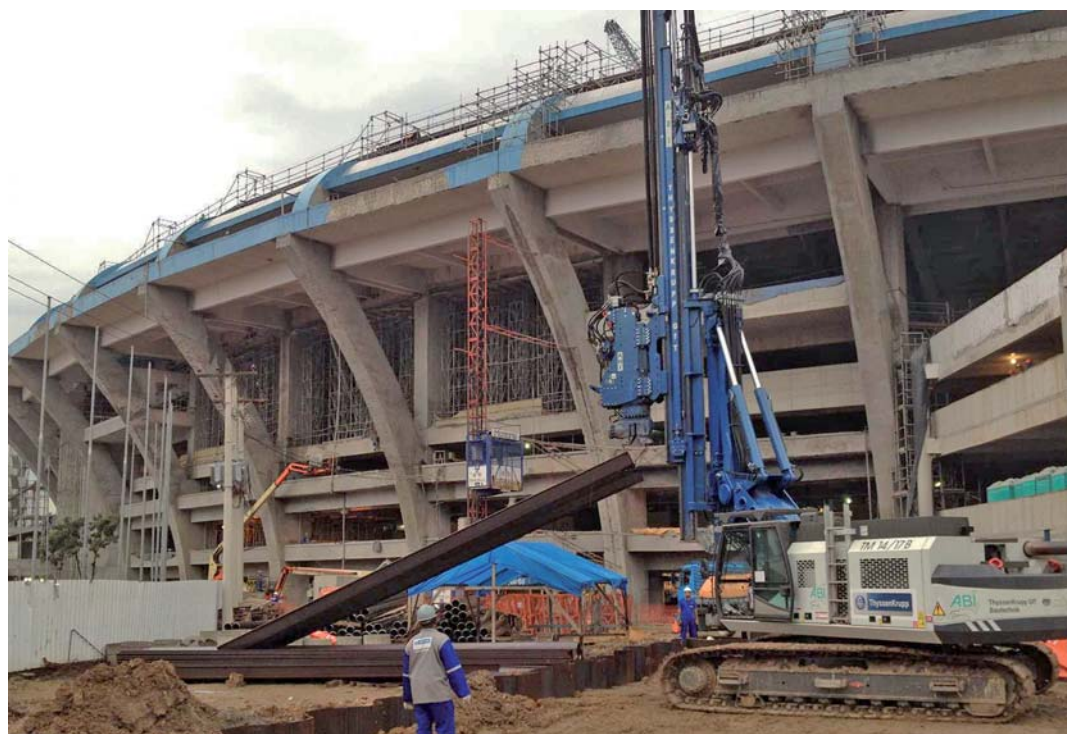
Photo above: Two ABI machines at Maracanã Stadium in Rio de Janeiro. The TM 18/22 B with auger drive MDBA 4000 pre-drills approx. one meter shorter than the pile length, the TM 20/25 with vibrator MRZV 36VV drives the double steel sheet piles to the required depth of 14 m.
