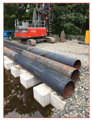
The 17 metre steel 'tree pole' piles were then inserted into the pre-auguered casing and vibrated further down resulting in them being approximately 12 metres below river bed level and standing 5 metres proud above normal river conditions.
