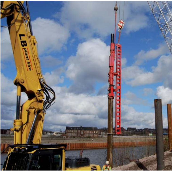
Photo: DELMAG diesel hammer D19 with swinging lead MS 1202 in Glasgow
