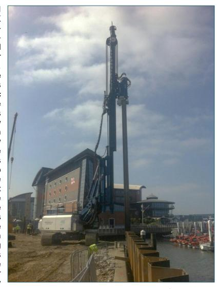
so with heavier piles and/or in more cohesive ground. The low total weight of the vibrator also means there is more capacity available to handle heavier piles, making the prospect of productively installing pairs of efficient sheet pile sections a reality.
