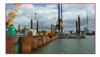
The contract stipulated that noise was to be kept to a minimum which precluded the use of noisy impact hammers driving the piles. This necessitated the use of a drilling rig to pre drill and install the piles.
