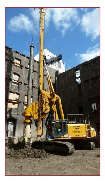
The Rig was used to construct a secant pile wall, consisting of 91 'hard' and 91 'soft' infill piles which were installed around the perimeter of the site. It was a very tight site where space was limited.
