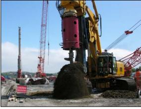
The contact involved the installation of bridge abutment and wing wall piles on the Heads of Valley A605 road widening project.
