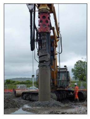
Stuart went on to say "this contract was very challenging with regard to the type of ground we were drilling. The 'piling rig grave yard' is one of the nick names for the area. Boring times varied between 3 hours and 2 days on piles that were adjacent to each other. We were changing teeth on augers and core barrels with each dig. We were very satisfied with the productivity and performance of the rig from ABI".
