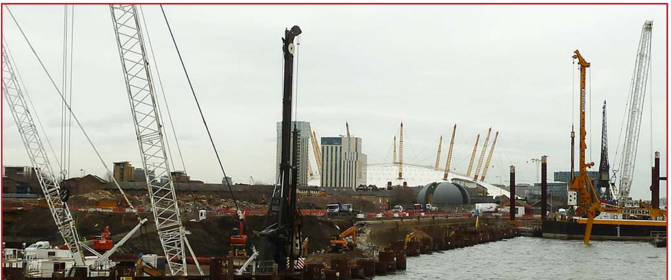
The combi-wall piles were installed by ABI's Delmag RH34 piling rig on a previous contract during the summer of 2015
