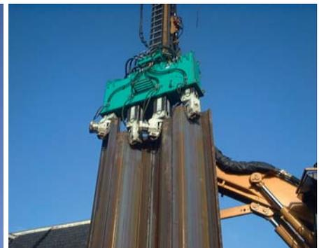
The pushing and pulling units (1) can be operated together in one step or separately from each other. Three or four clamp assemblies (2) with pitching chains (3) are mounted at the bottom of the Hydro-Press-System. Clamp assemblies are activated separately or together. In one movement the sheet piles are pitched, aligned and pressed as a panel driven/pushed into the soil.
