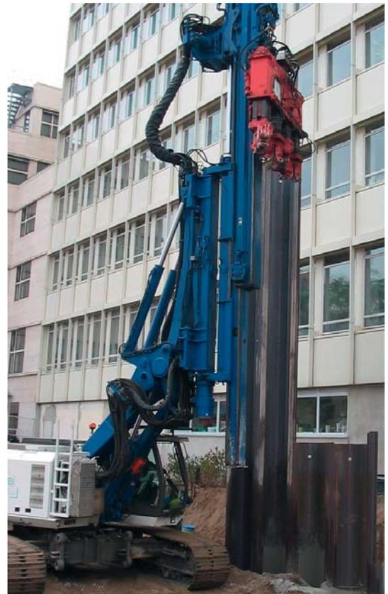
ABI offers three different types of Hydro-Press-System for various sheet pile types:
