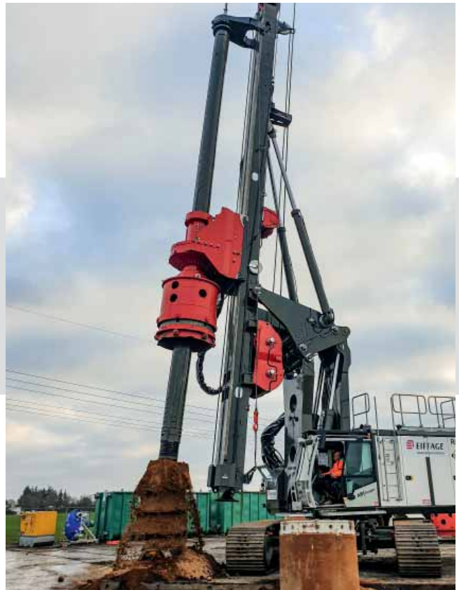
Drill rig with Kelly bar guide: In the case of inclined piles, the Kelly bar is also guided at the upper end to prevent the Kelly bar from tipping.
