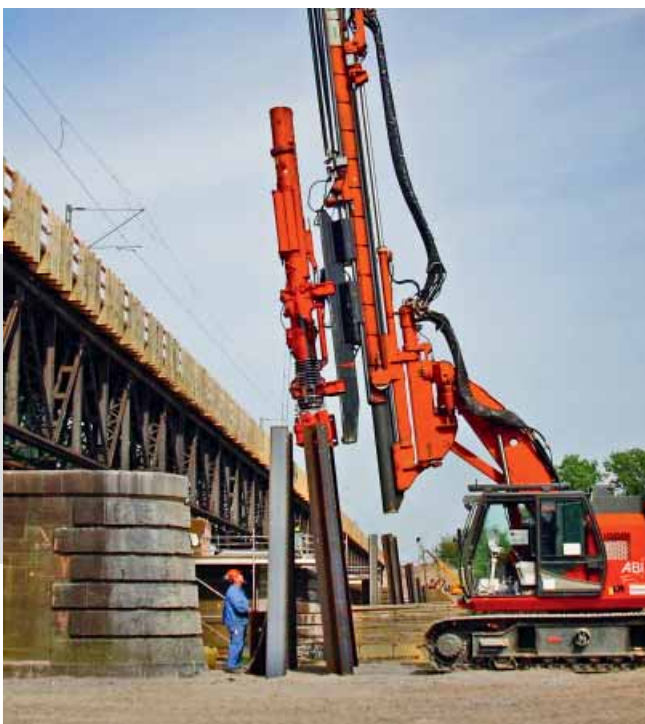
Impacting H-beams with DELMAG diesel pile hammer. With the DELMAG formula the load bearing capacity of the element can be calculated.
