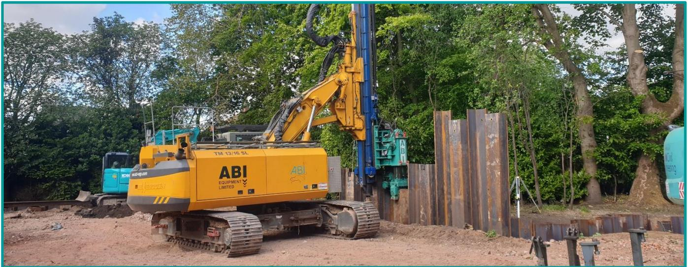
Due to the age and characteristics of the listed building it was decided to complete the final section of piling closest to the existing structure using a Mobilram HPU 600 Hydropress attachment. This method uses hydraulic power to press the piles into place rather than vibration – and is often called upon for use in the most sensitive areas.
