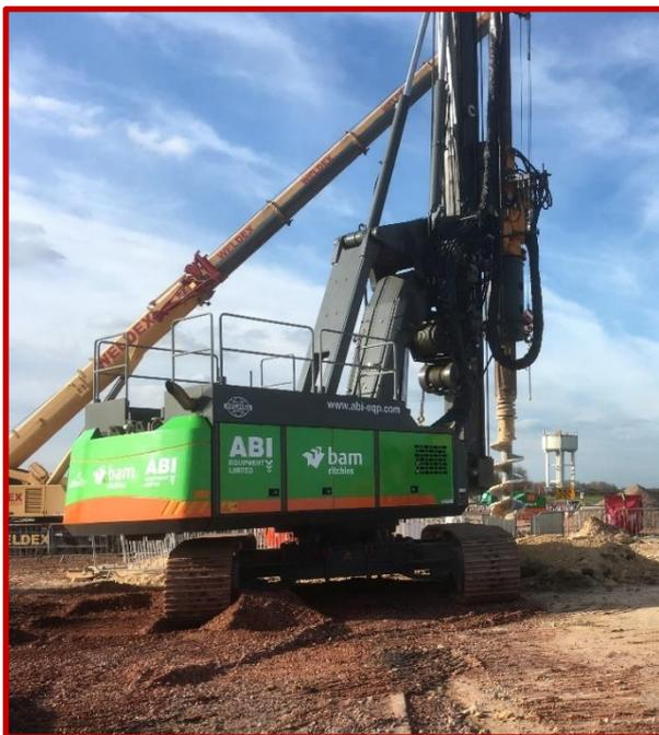
Limestone by its nature is extremely hard and tough, so a powerful rig was needed to execute this. Delmag rigs are renowned for their robust credentials – the RH28 offers 288 kNm of torque and 420kN of delivered crowd force in a rig that retains its mobility and agility on site – and so was highly suited to this job.
