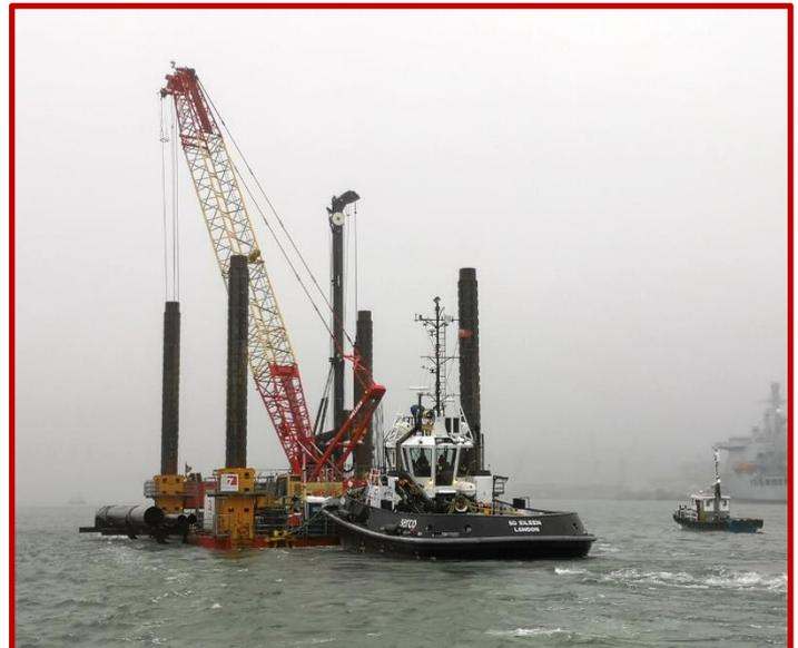
Two piles were required to be sunk, between which a 40m linkspan will land onto the new proposed pontoon structure. The pontoons will be fastened to the new piles to hold them in position. All work was carried out from Red7Marine's 400t jack-up barge sited just offshore in the tidal estuary.
