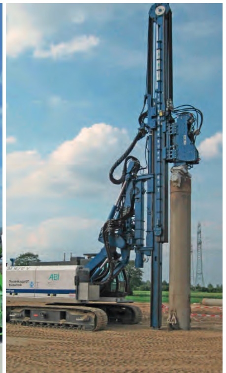
Installing geotextil piles: as a pile element a casing with reusable tip is used, after reaching the desired depth a fabric tube is inserted and filled with material.
