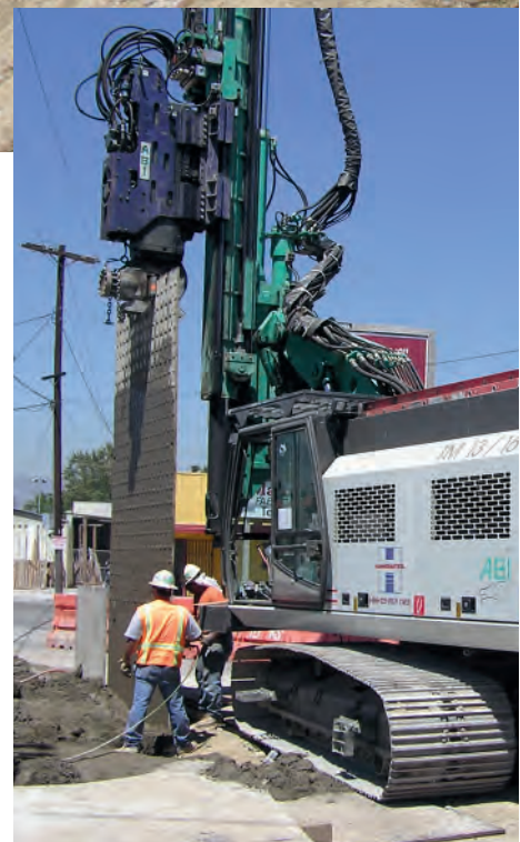
Driving large steel plates as excavation support.
