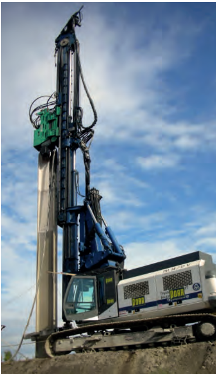
Installation of thin diaphragm wall as a sealing wall using a special H-beam. Displaced soil in form of the H-beam is filled with suspension.
