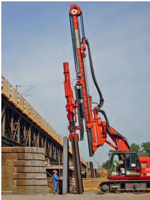
Impacting H-beams with DELMAG diesel pile hammer. With the DELMAG formula the load bearing capacity of the soil can be proved.
