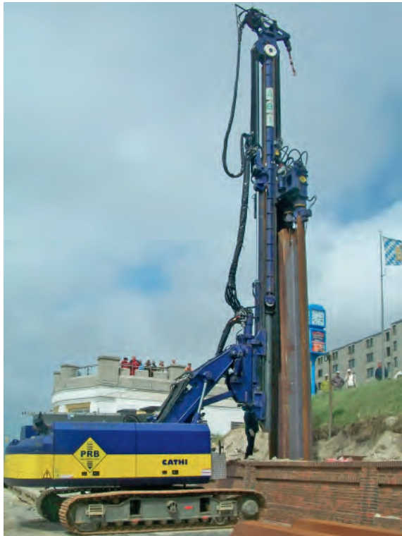
Static pressing with Hydro-Press-System: four steel sheet piles are pressed in a step sequence.
