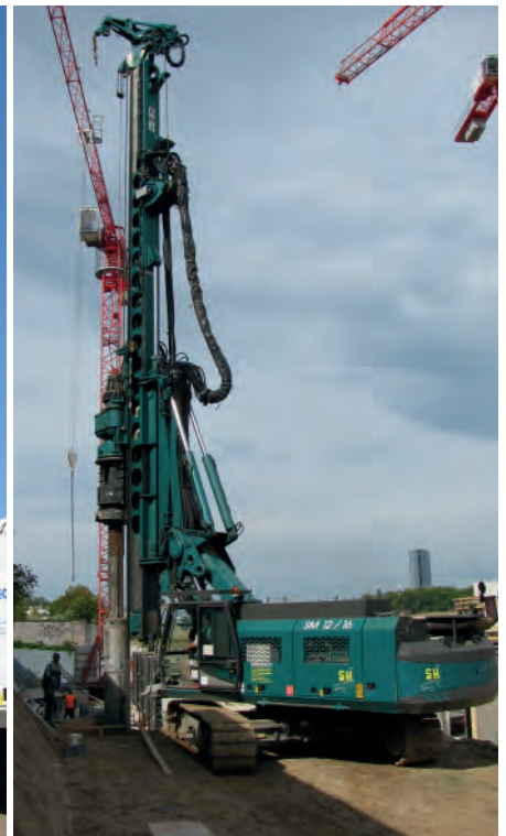
Kelly drilling: the machine is equipped with a Kelly winch. The casing is drilled as deep as possible first and then drilled out with the auger. This process is being repeated till the requested depth is achieved.
