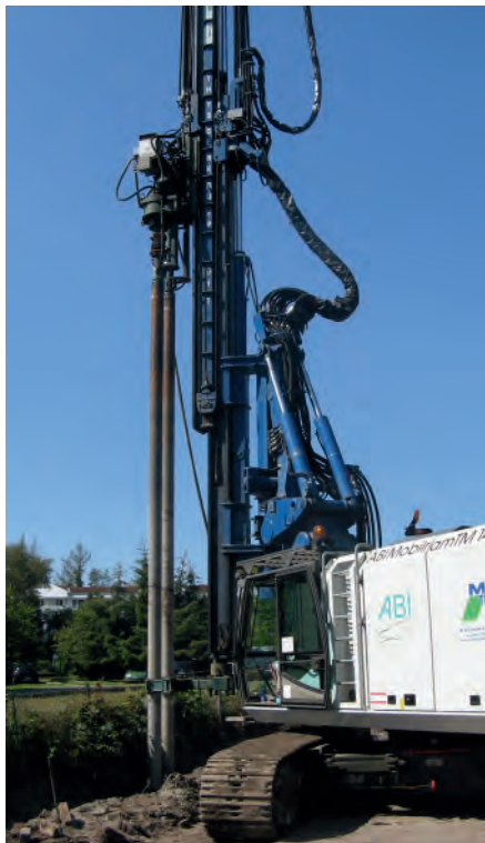
To achieve more efficiency the soilmixing procedure can be carried out as twin- or triplemix version, mixing two or three piles simultaneously.
