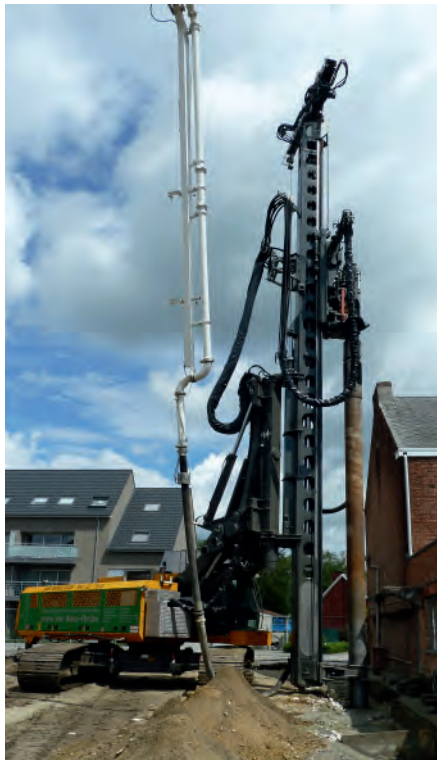
VDW drilling: the classic case of use - installing secant pile wall directly in front of existing structure.
