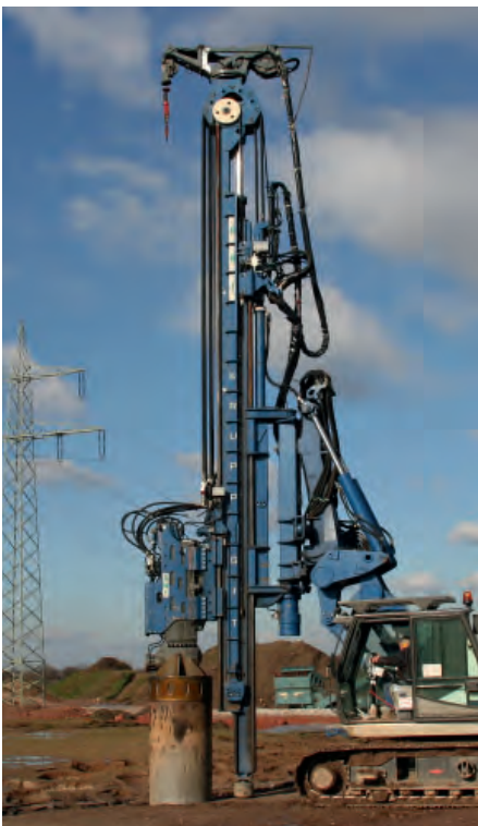
Soil improvement measure: large diameter casing is driven into the ground the resulting hollow space is filled with additional material.
