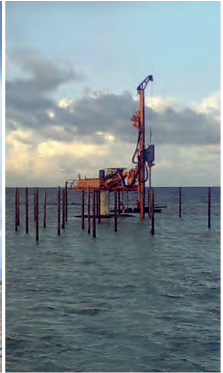
ABI groyne piling machine - between the crawler and upper carriage an intermediate piece (pylon) is mounted, so that the machine can be used for pile driving in shallow waters.
