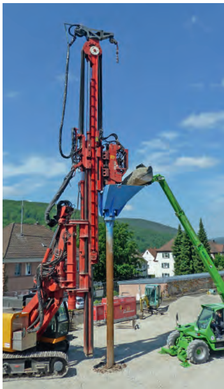
Stone columns: probe is driven to desired depth and while extracting the hollow space is filled and compacted with gravel using the pilger process.
