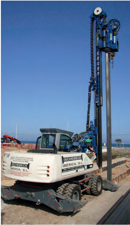
ABI MOBILTRAM TM 8/10 mounted on a wheel drive under carriage is particularly agile and flexible.
