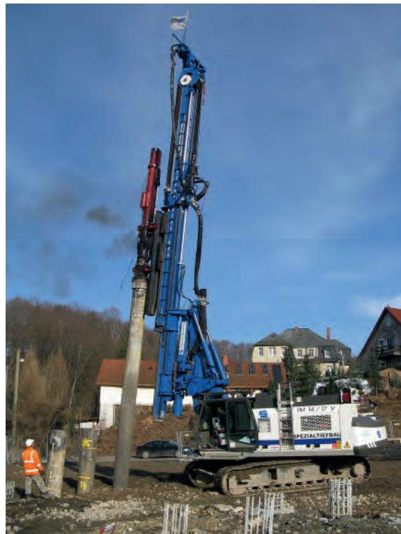
Driving casings with DELMAG diesel pile hammer.
