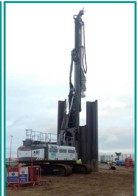
meant that the vibration frequency could be adjusted, and therefore what could have been potentially harmful resonance would be minimised.
