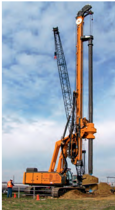
Uncased Kelly drilling
