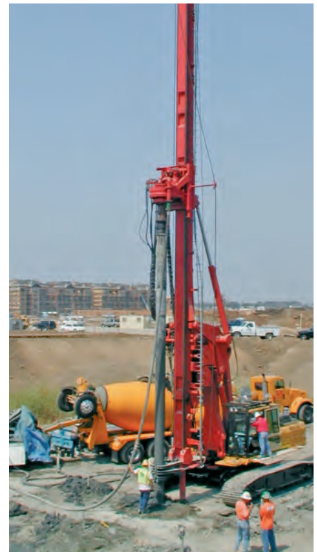
Full displacement drilling
