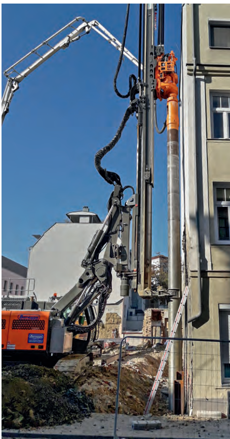
Photos: TM 17 with VDW 10050 at the job site Vivenotgasse, Vienna, finished building pit with secant pile wall and soldier beam wall (above)
