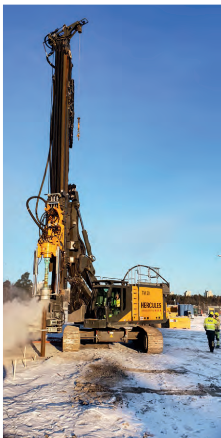
Photos: TM 20 with auger drive MDBA 3200 while DTH drilling (left and below)
