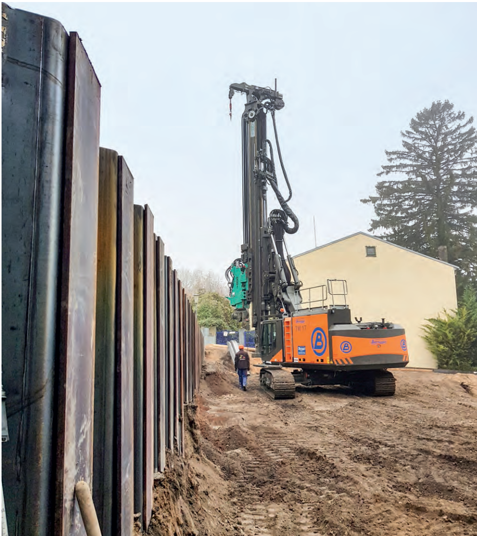
Photo: TM 17 with vibrator MRZV 20VV in the town of Bad Vöslau (left)
