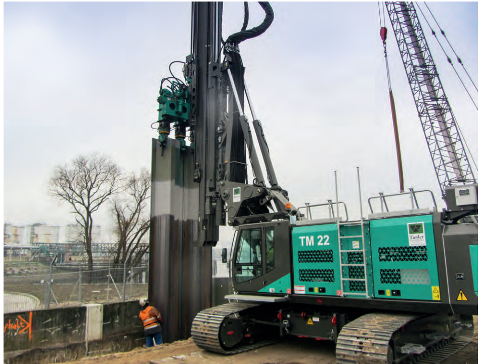
Photos: TM 22 with Hydro-Press-System (above), finished, coated steel sheet pile wall with steel sleeper (below)
