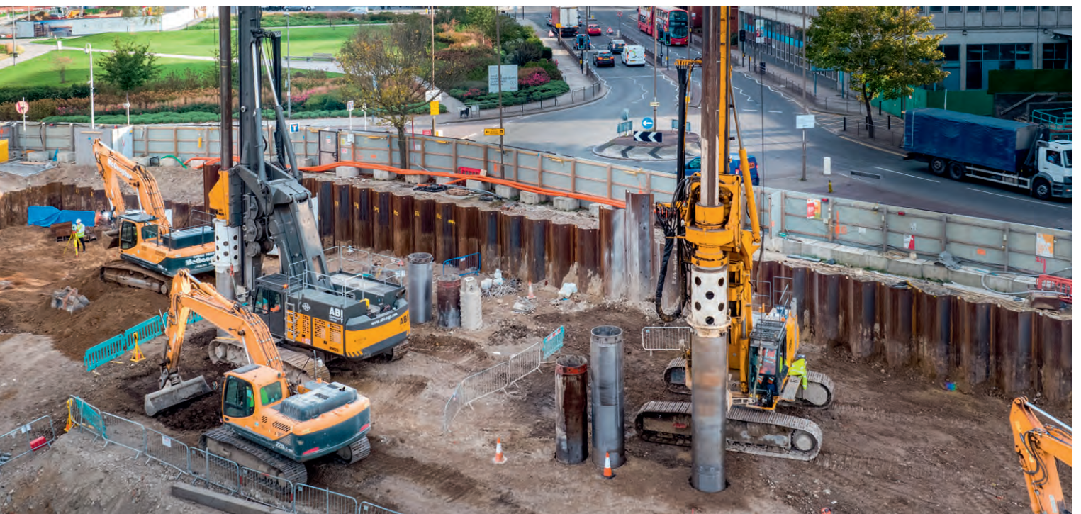
Photo: DELMAG drill rigs RH 28 in London on the Woolwich Royal Arsenal job site
