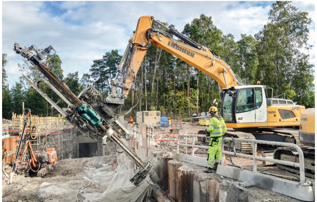
Photo: Anchor drilling with SPD machine DM55.2
