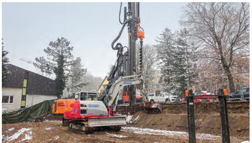
Photo: TM 17 with auger drive MDBA while pre-drilling in the town of Bad Vöslau
