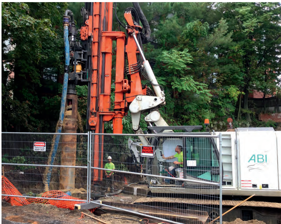
Photo: ABI MOBILRAM TM 14/17 V with VDW double auger head system
