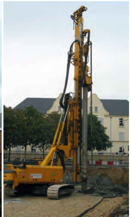
Double auger head system DH 18: works similar as VDW, but the auger heads are separately moveable. It enables the auger to be withdrawn while the casing is staying in the ground.
