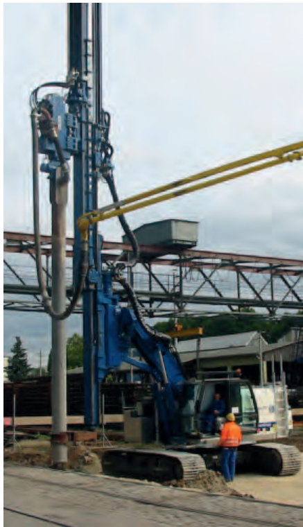
With a vibrator also full displacement piles with lost plate or reusable tip can be installed.
