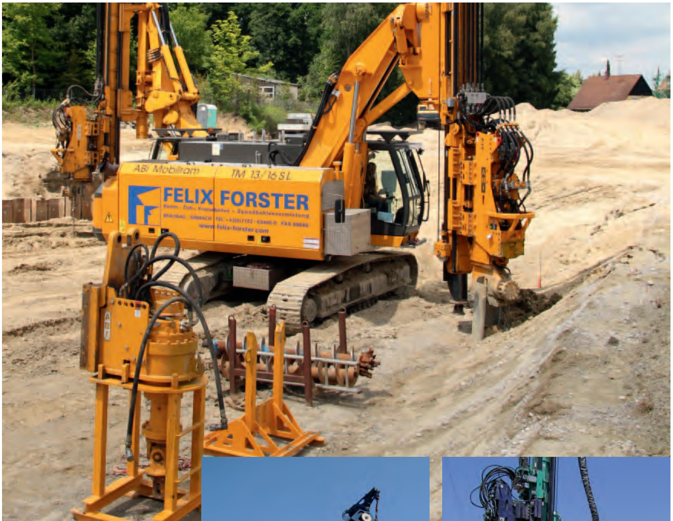
The classic case of use: driving steel sheet piles.
