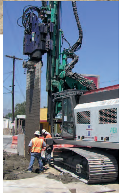
Driving large steel plates as excavation support.
