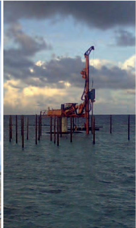
ABI groyne piling machine - between the crawler and upper carriage an intermediate piece (pylon) is mounted, so that the machine can be used for pile driving in shallow waters.
