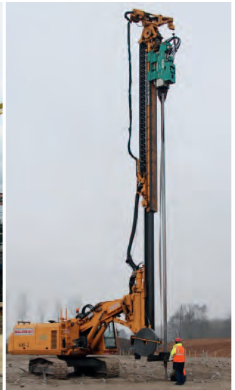
Installing wick drains in a tight pattern for water level control.
