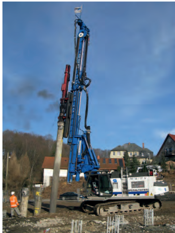
Driving casings with DELMAG diesel pile hammer.
