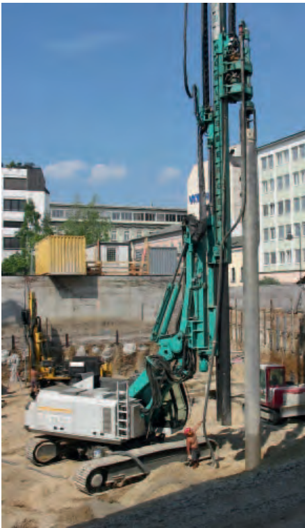
VDW drilling: with the VDW double auger head system cased single piles as well as secant pile walls can be installed. The drilling is carried out in one step, after drilling down concrete is pumped during withdrawal.
