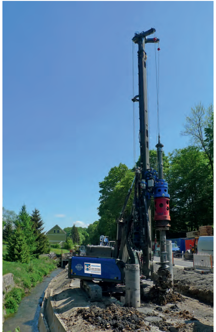
Photo: RH 12/140 of the company Hoch- und Tiefbau Reichenbach, construction number 2, while Kelly drilling along the creek of Wildenfels, Germany
