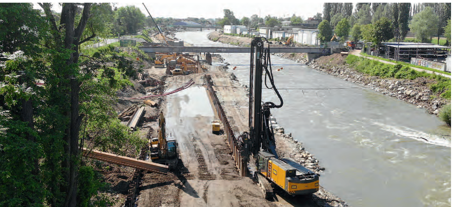
Photo: Ongoing site work at Central storage sewer in Graz
