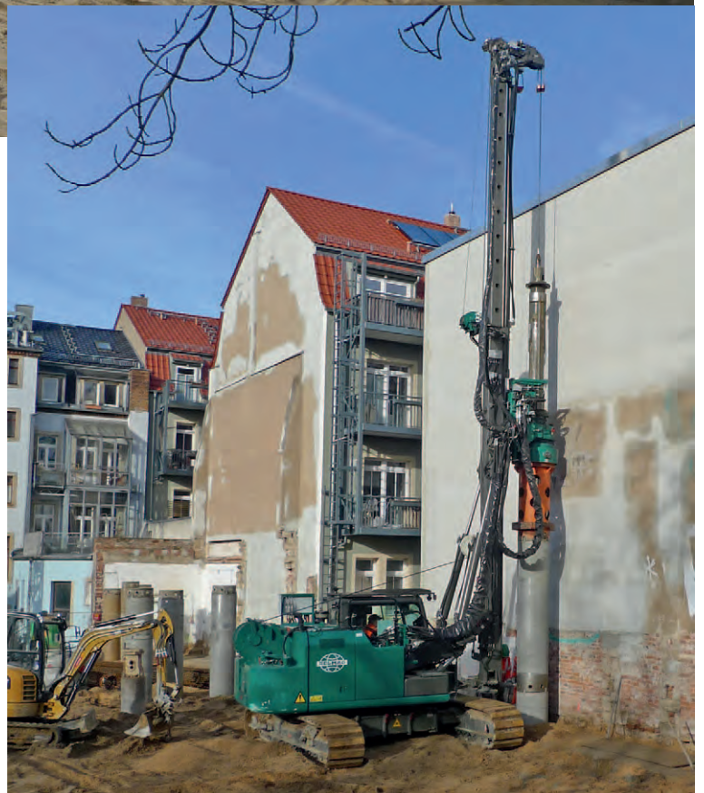
Photo: Finished secant pile wall and DELMAG drill rig RH 06 while drilling in Dresden
