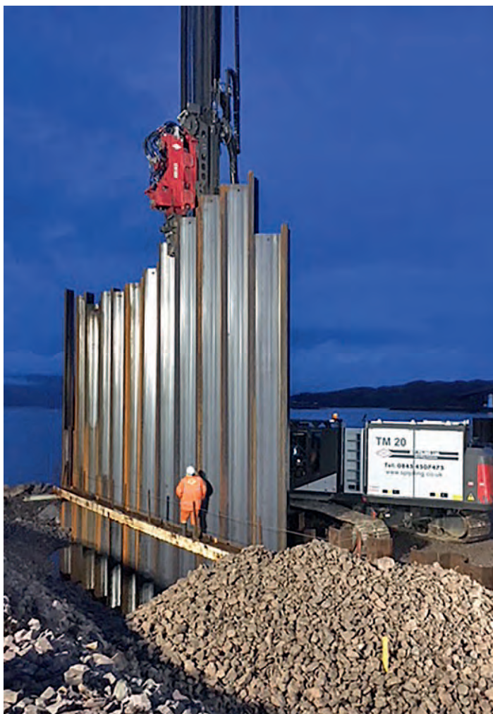
Photos: ABI combi clamp assembly MZK 1200 mounted on vibrator MRZV 30VV (above) Piling works with TM 20 in Kyleakin, Scotland (left)
