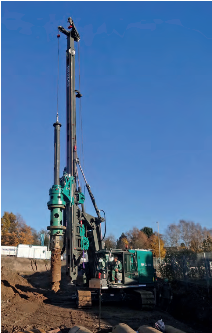
Photo: RH 12/140 of the company S+H Spezialtiefbau, construction number 1, with rotary head BT 140 in Bonn-Beul, Germany while spinning-off the soil
