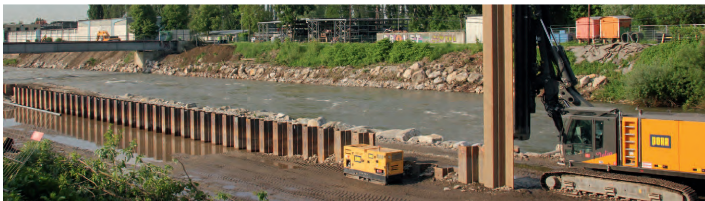
Photo: ABI MOBILRAM TM 20 at the river of Mur in Graz, Austria
