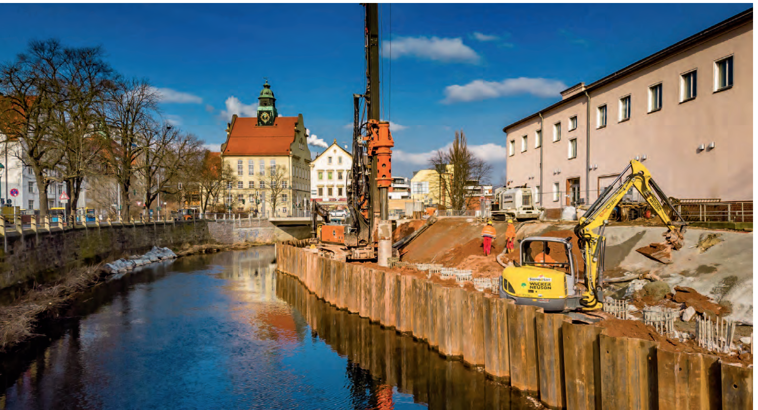
Photo: DELMAG drill rig RH 24/270 of the rental fleet of the company BWH Bohrwerkzeuge Hoffmann working in the centre of Chemnitz, Germany
