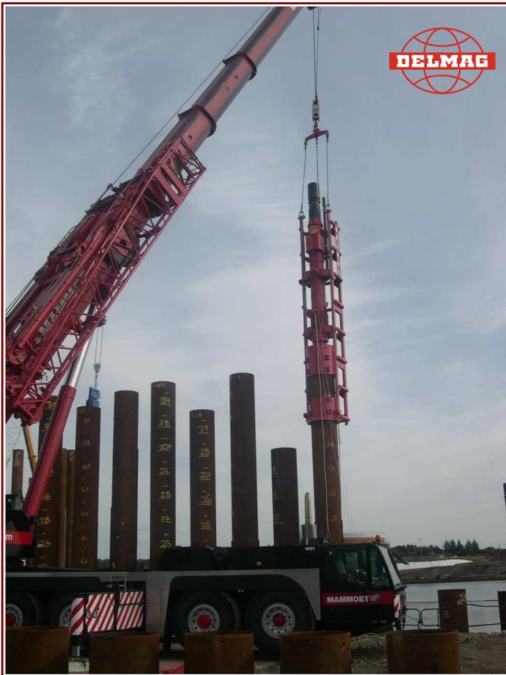
Delmag hammers can be equipped with a hydraulic starting mechanism where they may be used with hydraulic piling rigs, for example.
