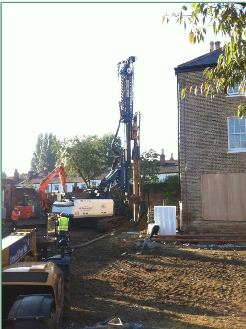
Concrete secant piles were installed, primarily in clay soil conditions, around the perimeter of this development to form a basement and swimming pool area. The job required the installation of 318 No x Ø420mm piles to depths between 8 and 12m, with a maximum retained height of 8m.
